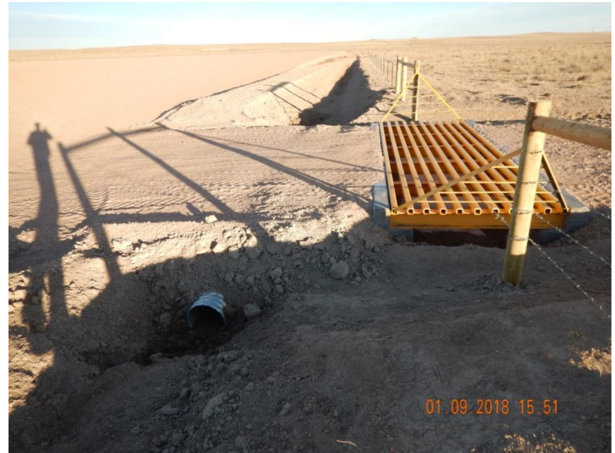
Photo 4. Photo taken from the southern location, facing East. Vehicle tracking device installed. Culvert installed in conjunction with the ditch BMP.
