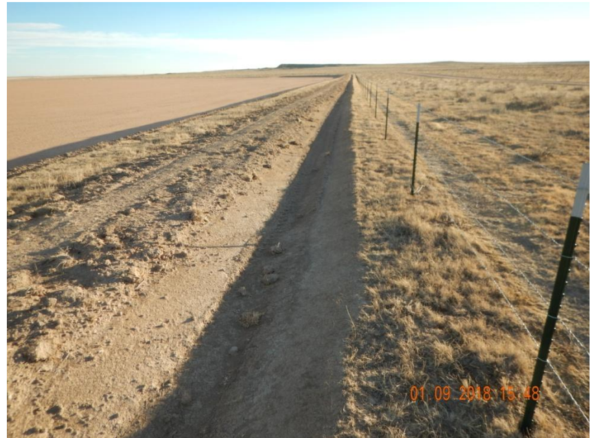
Photo 2. Photo taken from the western location, facing South. A ditch BMP has been installed along the perimeter location.
