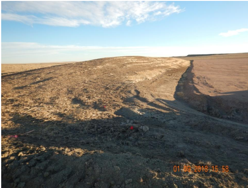
Photo 7. Photo taken from the northeast location, facing South towards the topsoil stockpile. Photo illustrates portions of the topsoil are bare and may require additional stabilization.
