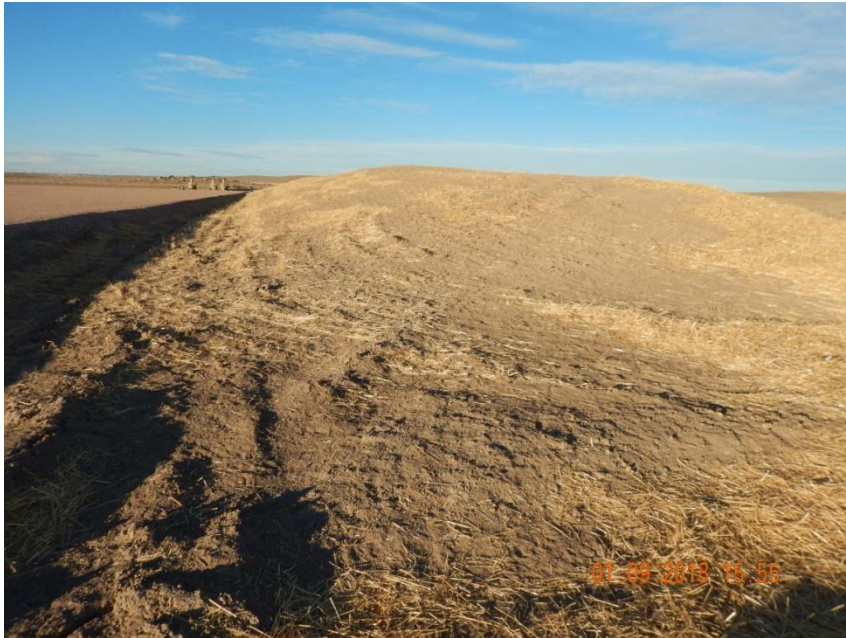
Photo 5. Photo taken from the eastern location, facing North toward the topsoil stockpile. Straw mulch is blowing off topsoil which may need maintenance.
