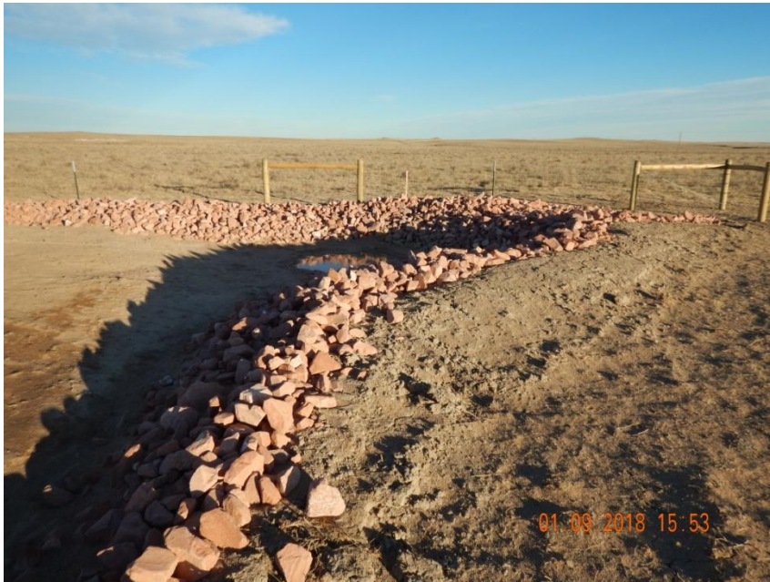
Photo 1. Photo taken from the southeast location, facing East. A sediment trap with a stabilized outlet has been installed. Operator may want to consider an additional sediment trap as this is the only sediment trap for a total disturbance of 19.17 acres which will not be reclaimed to reduce the total disturbance for interim reclamation.
