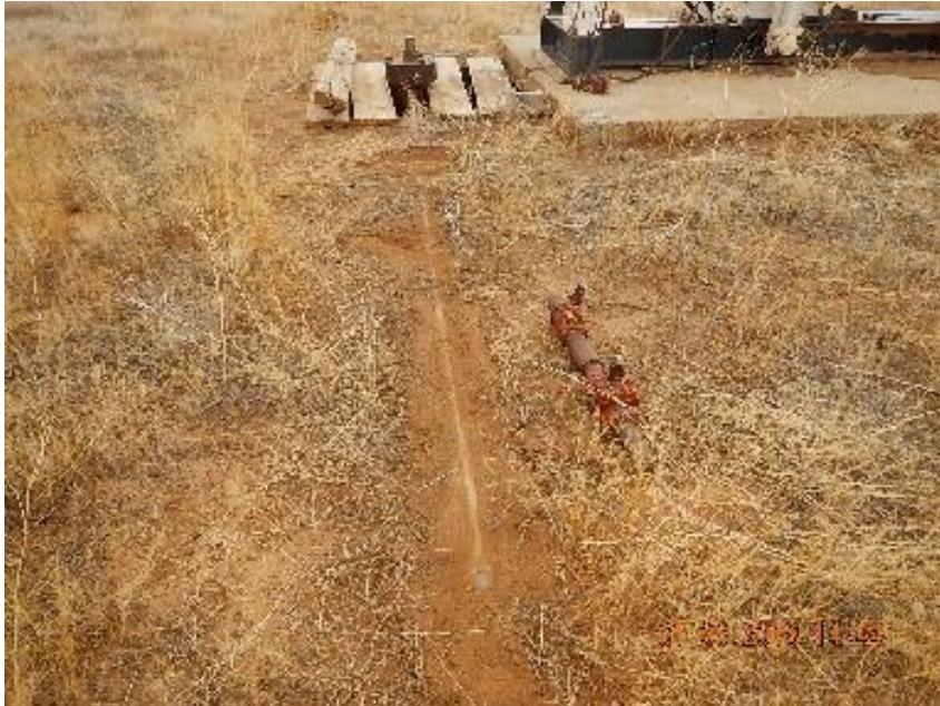
Photo 3: Flowline from wellhead and steel riser out from wellhead.
