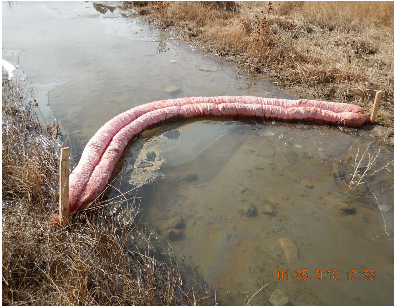
Wet Canyon just below dry drainage where spill was sourced. Booms in place.
