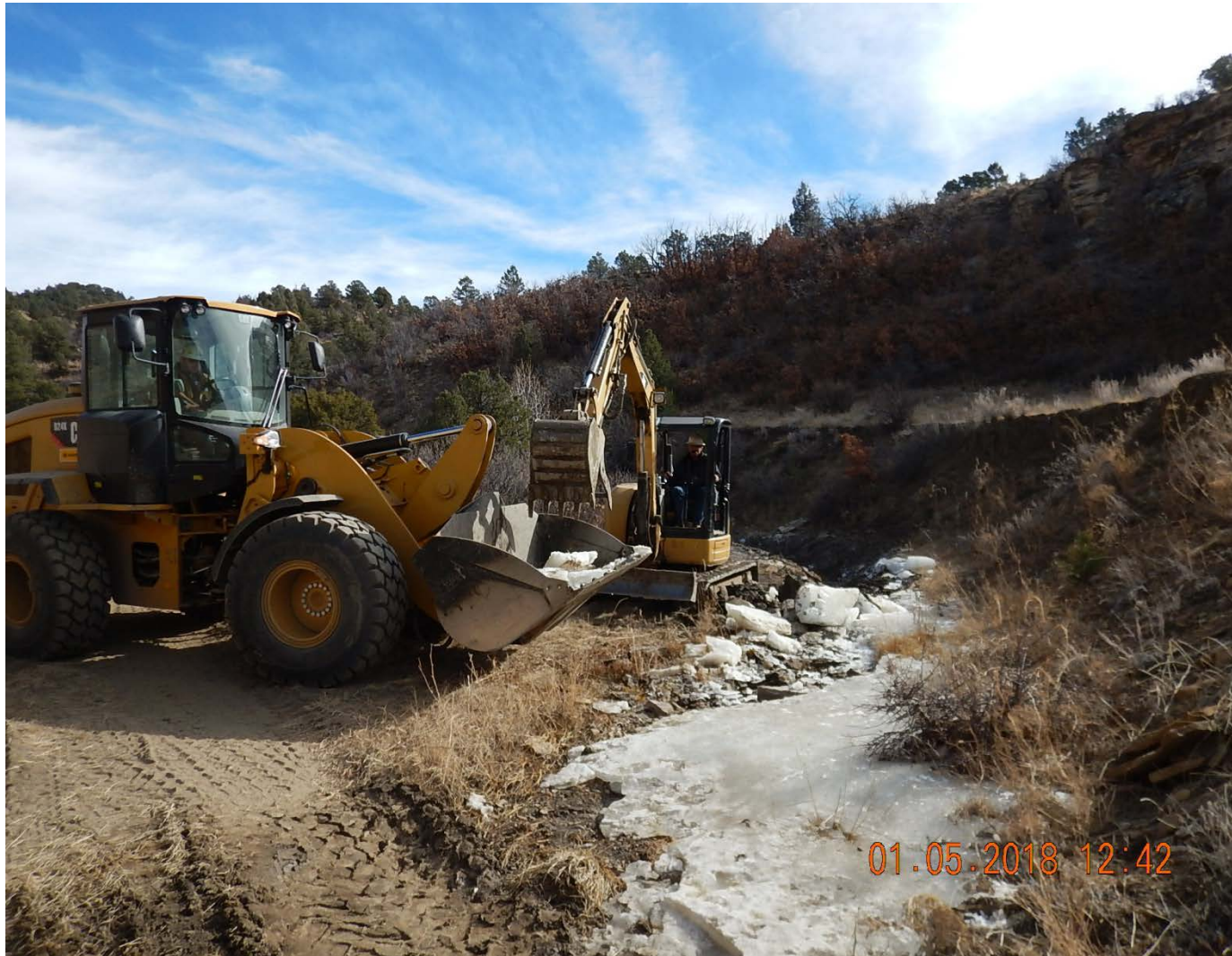
Dry drainage below spill source. Frozen spilled material being removed.
