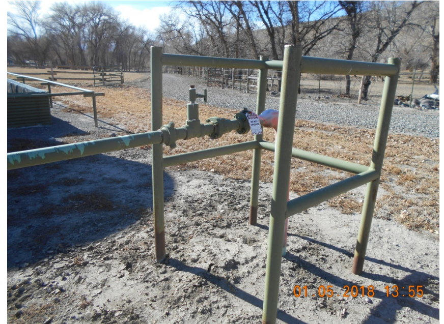
Flowline riser marked locked out / tagged out.
