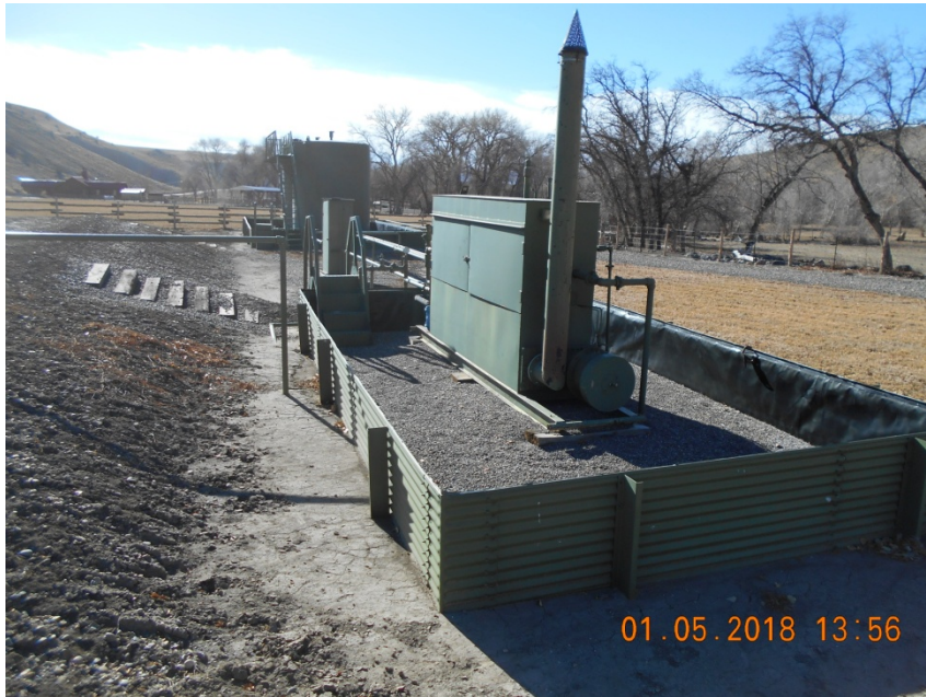
Separator and tanks with metal berms.
