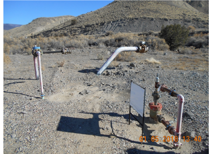
Flowline risers Marked/locked out tagged out.
