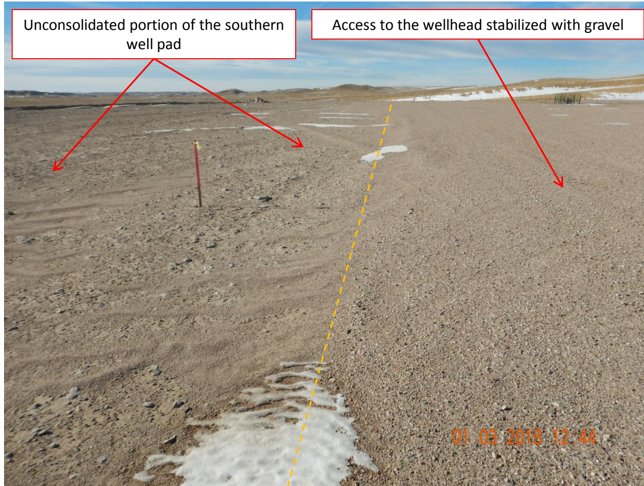
Photo 1. Photo taken from the east central well pad, facing West on January 3, 2018. Sediment discharge off location is evident due to wind erosion from unconsolidated soil material from the well pad. Operator has only stabilized a portion of the well pad with gravel for access to the wellhead and around the wellhead. All other areas of the well pad have been left unconsolidated which appear to be the cause of wind erosion off location.
