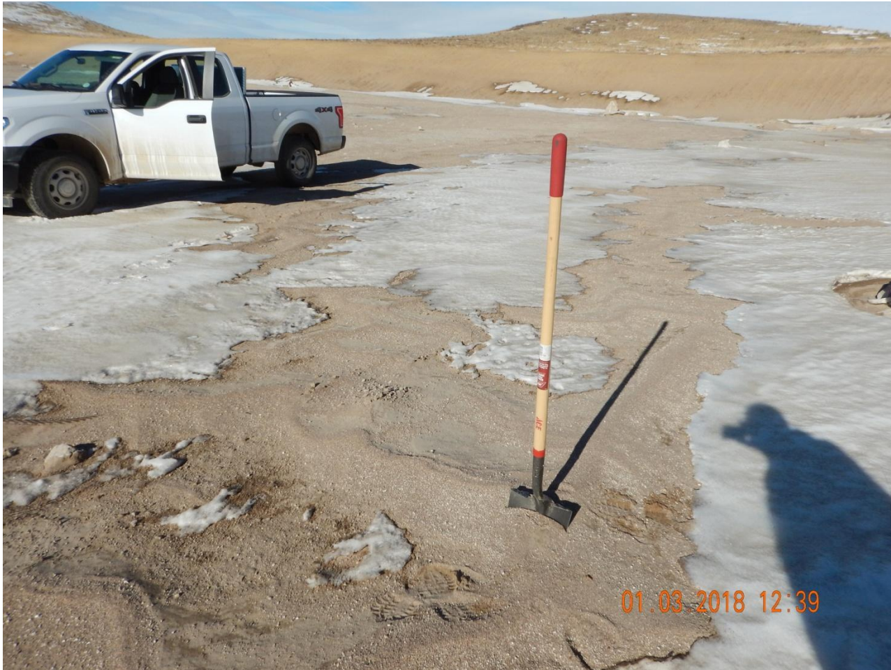
Photo 7. Photo taken from the east well pad, facing North on January 3, 2018. Photo illustrates accumulation of unconsolidated soil material from the well pad which is contributing to sediment discharge off location.
