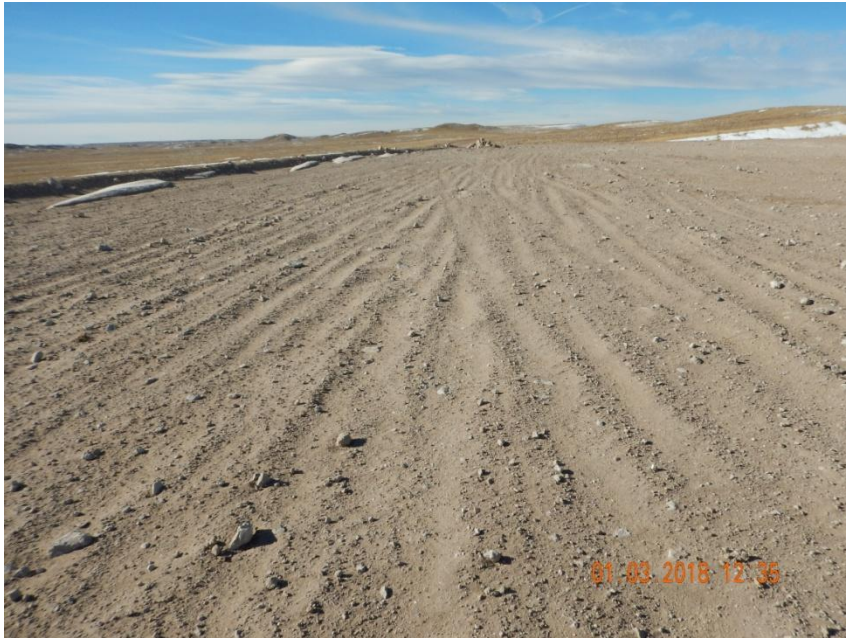
Photo 2. Photo taken from the southern well pad, facing West on January 3, 2018. The southern and northern well pad areas have not been stabilized and left unconsolidated which appears to be the cause of wind erosion off location.
