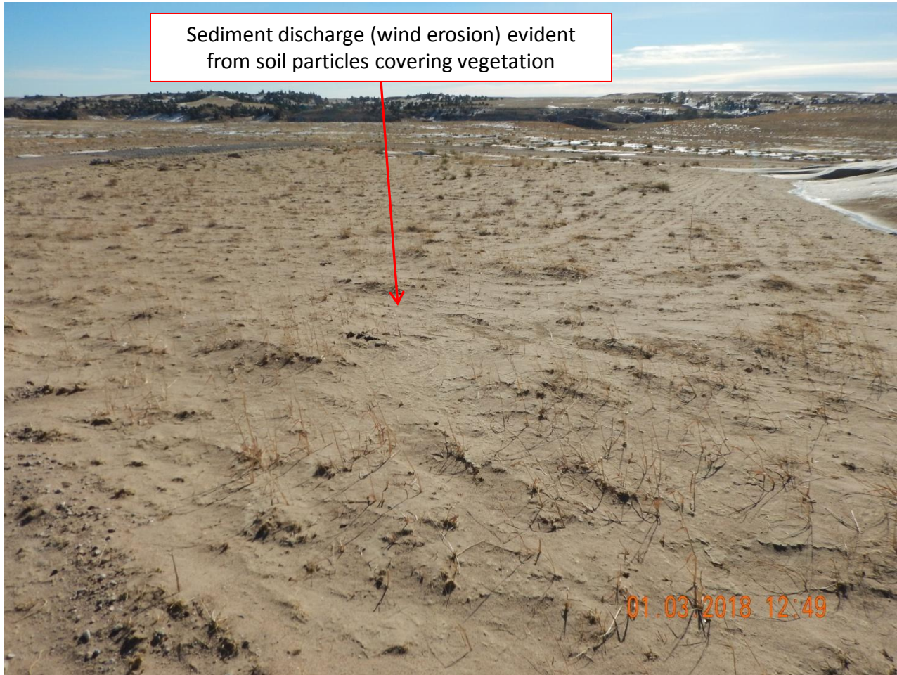
Photo 16. Photo taken from the eastern location on the fill slope, facing Southeast on January 3, 2018. See comments under Photo 9.
