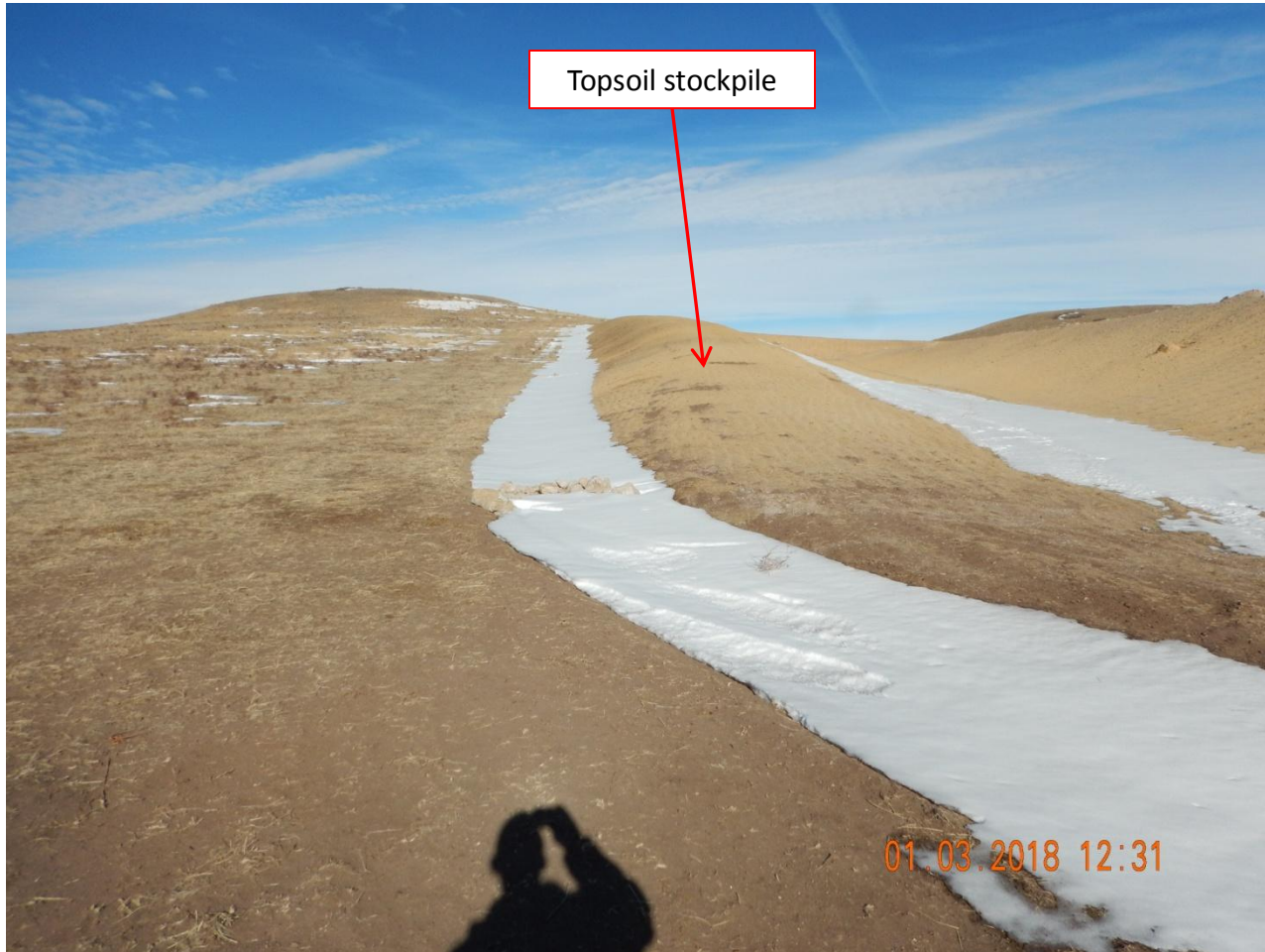
Photo 11. Photo taken from the southwest location, facing North on January 3, 2018. Since the October inspection, it appears the Operator has installed a perimeter ditch along the outer perimeter of the location in conjunction with check dams (rip-rap) and applied a hydromulch to the topsoil stockpile, fill and cut slopes.
