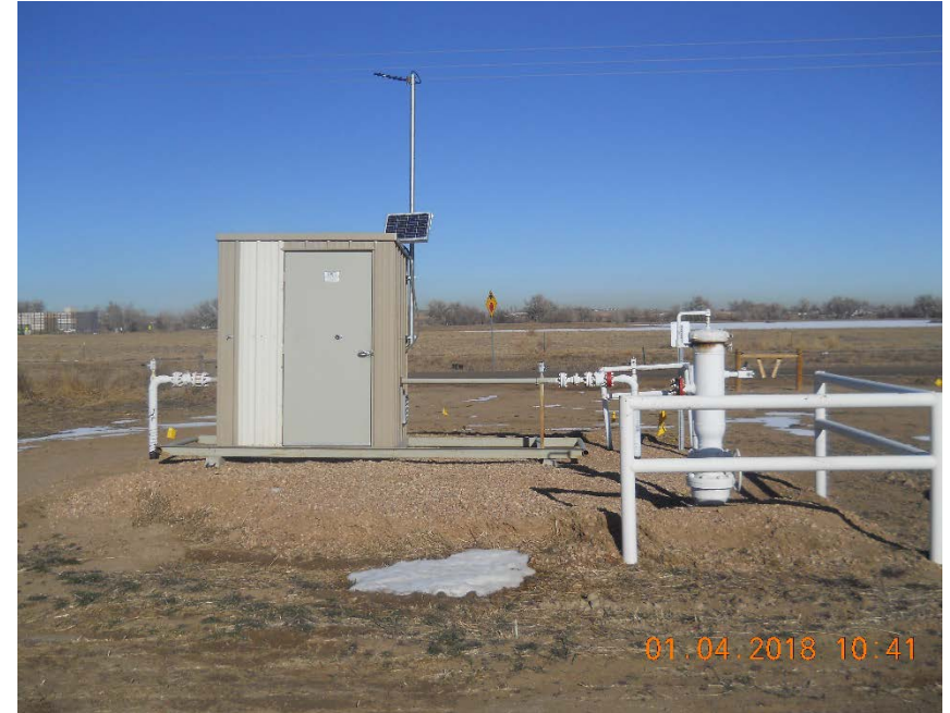
Gas meter run and pig launcher are still in place. Gas meter run is still connected upstream and downstream. Upstream riser possibly buried and capped. Photo taken at 40.43969, -104.83016 looking north
