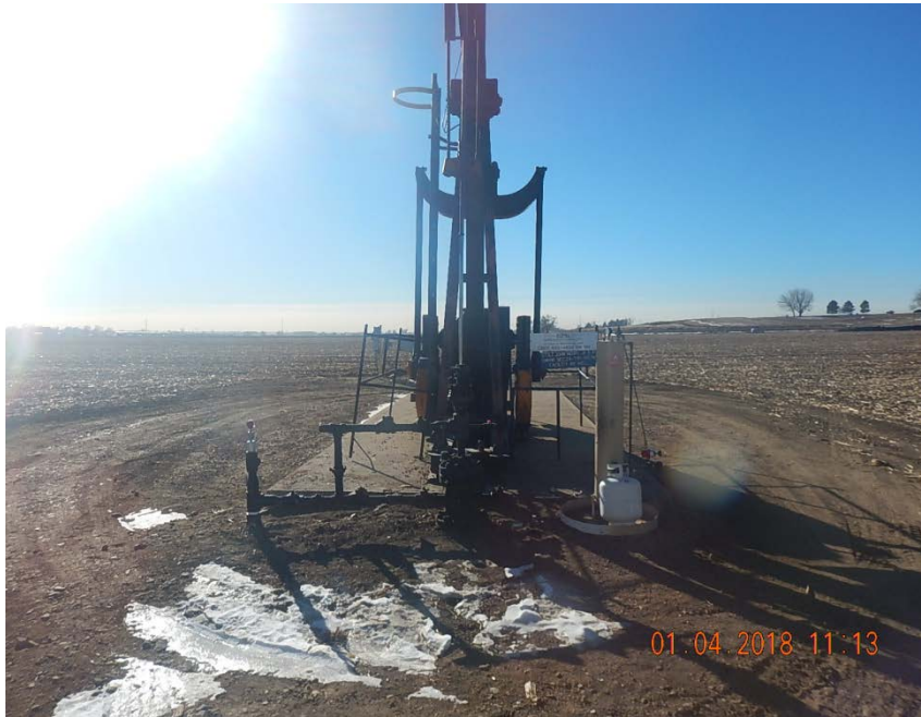
Photo 1: Wellhead, looking S
