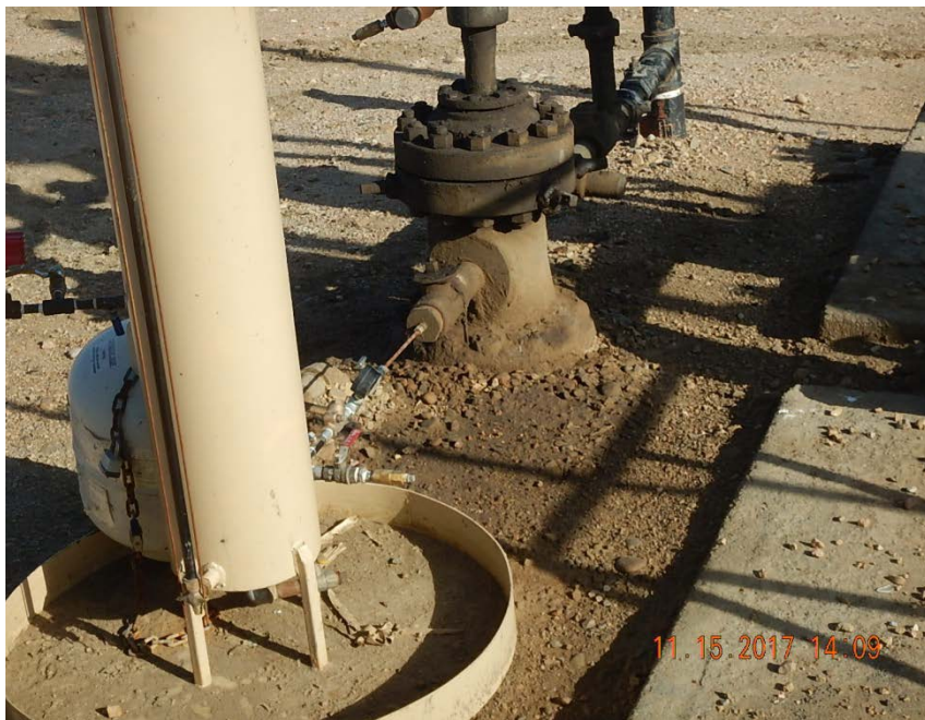
Photo from prior inspection for comparison
