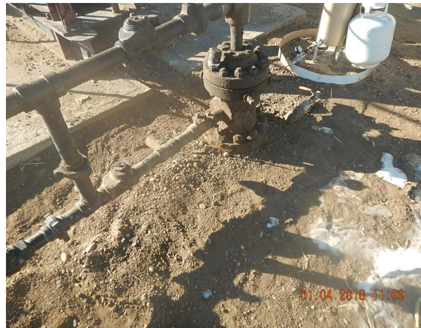
Photo 2: Stained soil removed
