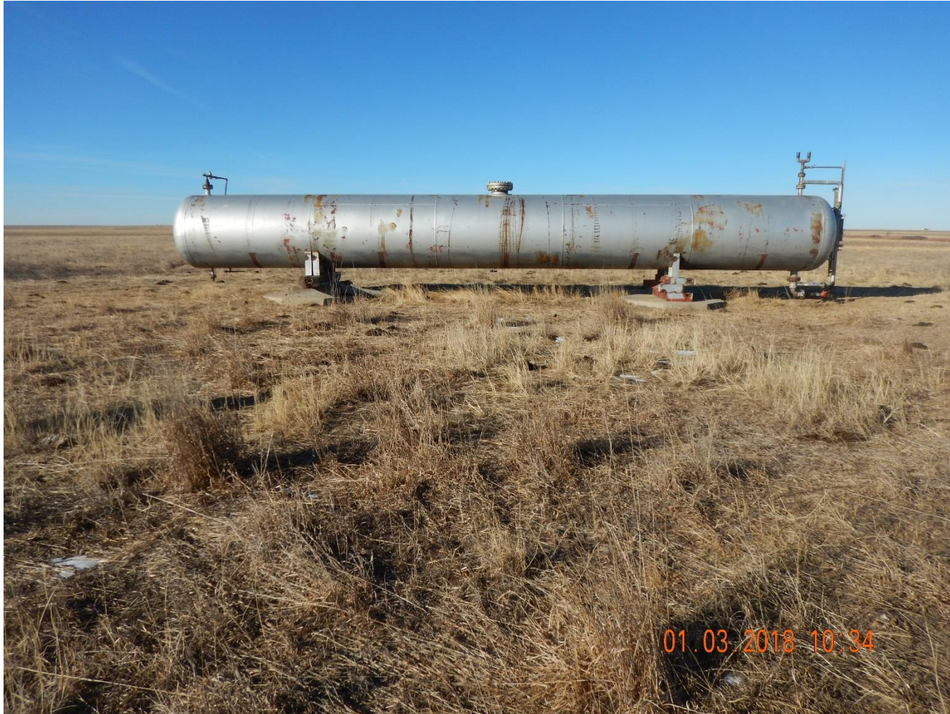
Photo 7: Photo taken from the north end of the location, facing west. Photo shows a ~50 foot “Propane Storage Tank” remaining on the location. Equipment should have been removed in accordance to 1004.a. COAs for form 27 #2086957 also required removal of equipment.
