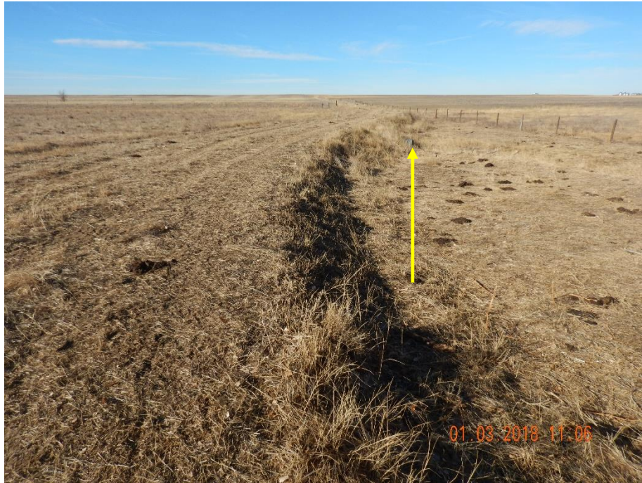
Photo 16: Photo taken from access road, north of the location, facing west. Photo shows access road has not been reclaimed and culverts (yellow arrow) have not been removed.
