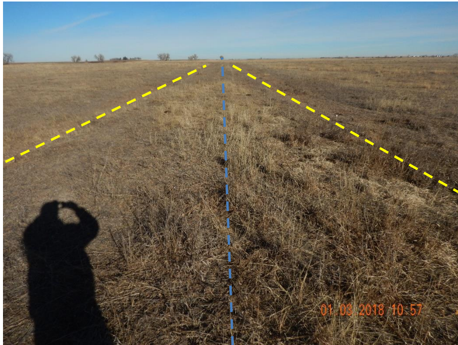
Photo 10: Photo taken from the north end of the location, facing north. Photo shows access road has not been reclaimed in accordance to COGCC 1004.a reclamation requirements. Access road appears to be requiring grading and re-contouring to that of the adjacent reference area. Yellow lines indicate the access road's stormwater ditch running parallel to the road (blue line represents top of access road)
