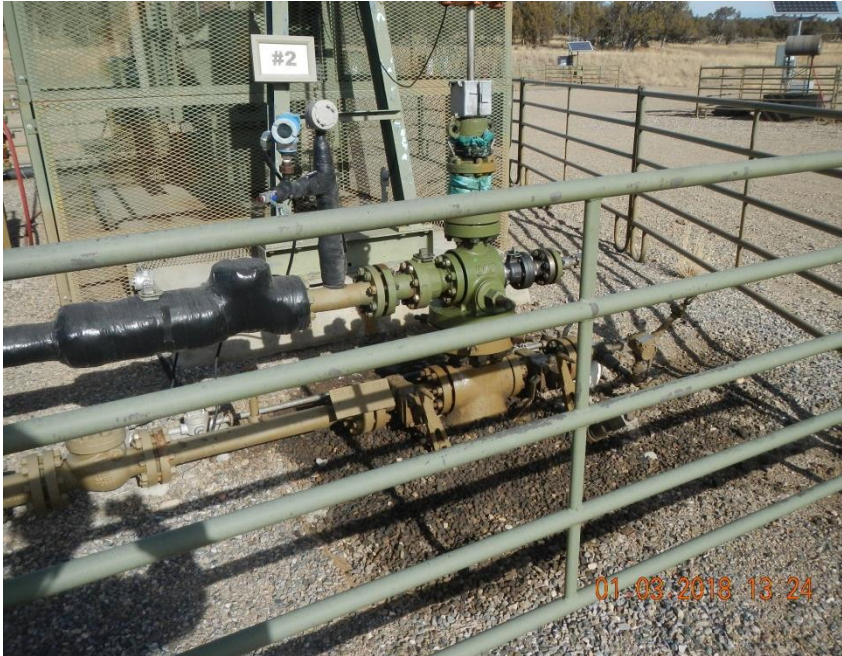
Stained soil around #2 well head. Absorbent rags tied to well head are saturated.
