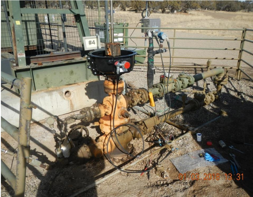
BP representative on site installing a float controlled trap.
