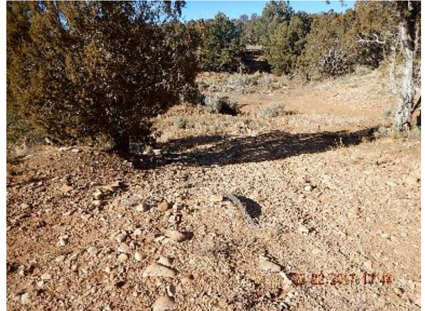
Photo 12: Line popping above ground along access road at top of drainage.
