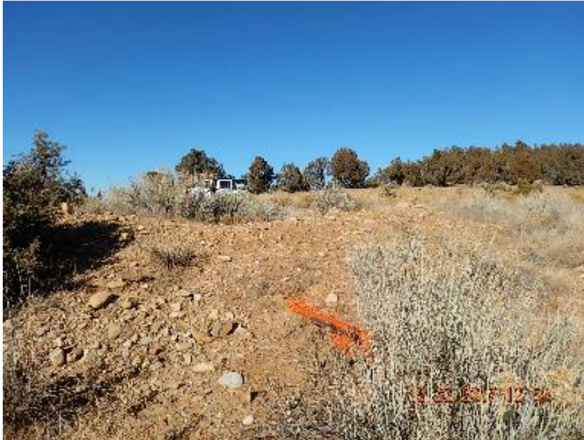
Photo 5: Exposed flowline coming out of slope on the SE side of location.
