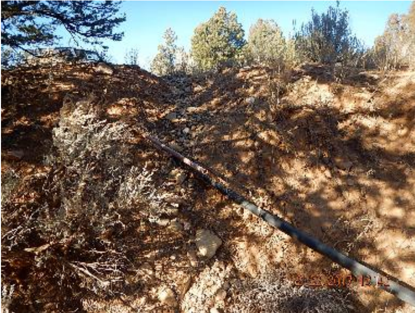
Photo 9: Exposed lines at washed out area on access road.
