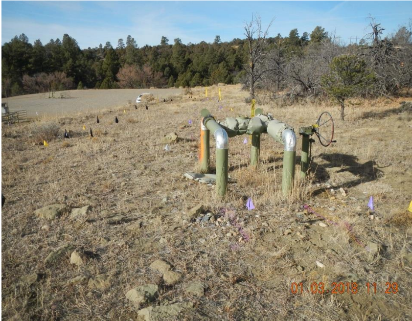
Pipeline risers north of well pad.
