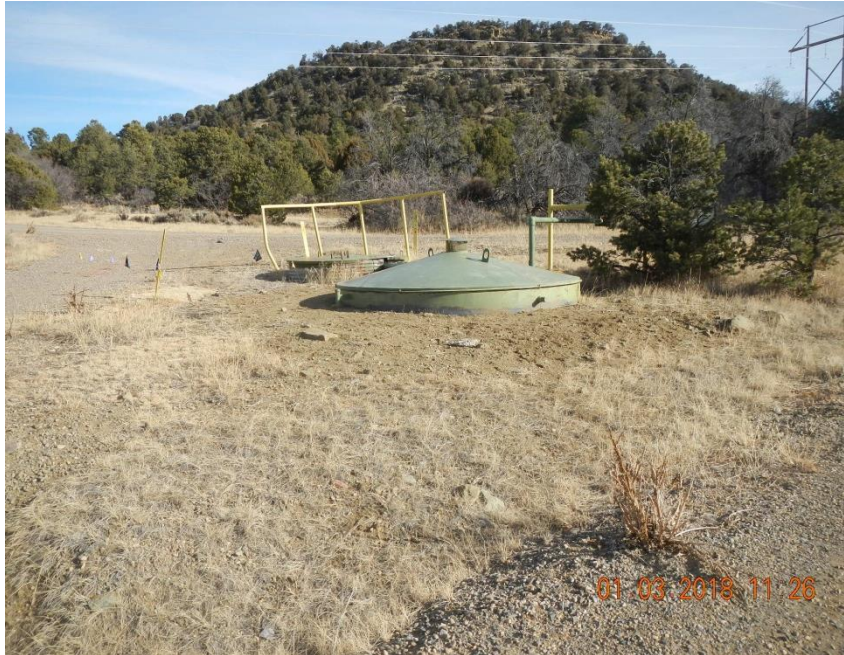
95 bbl. PBV without secondary containment.
