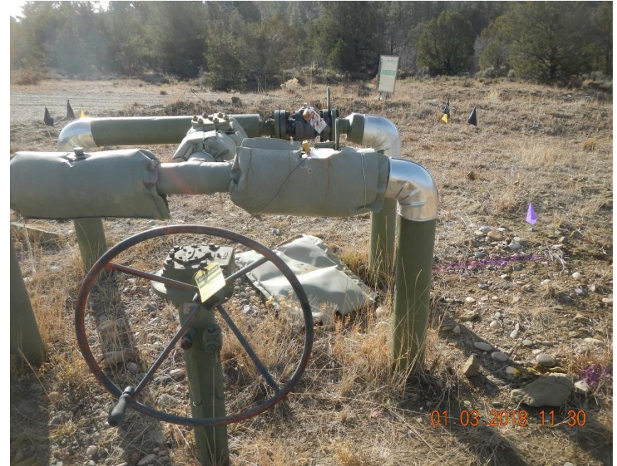
Valves are locked out on risers.
