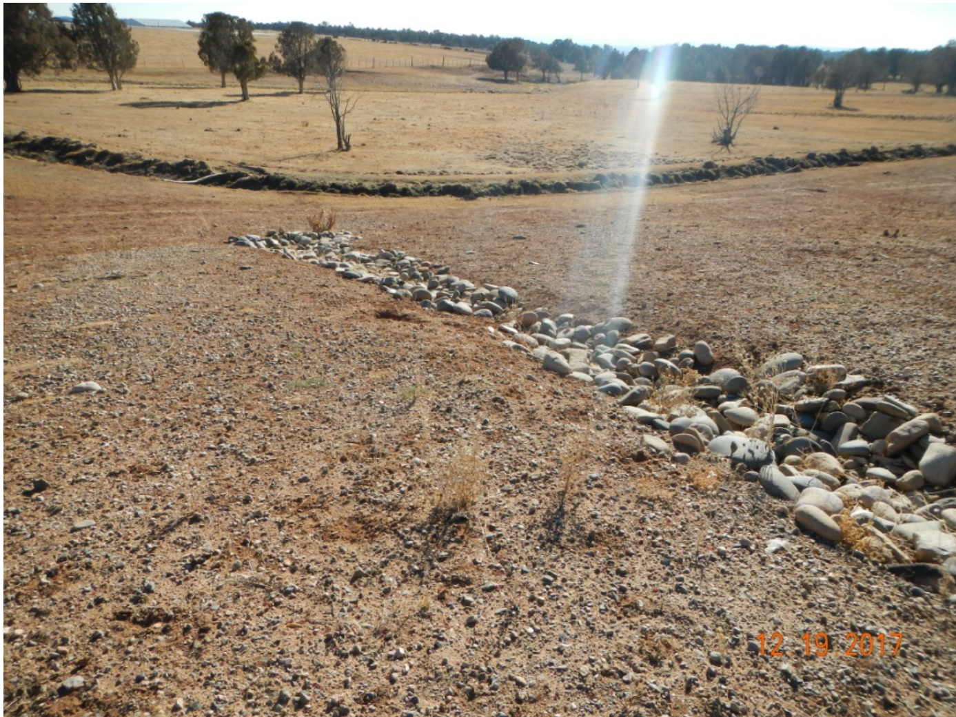
Photo 4. View of stormwater controls in the southern portion of the project area, appear to be functioning.
