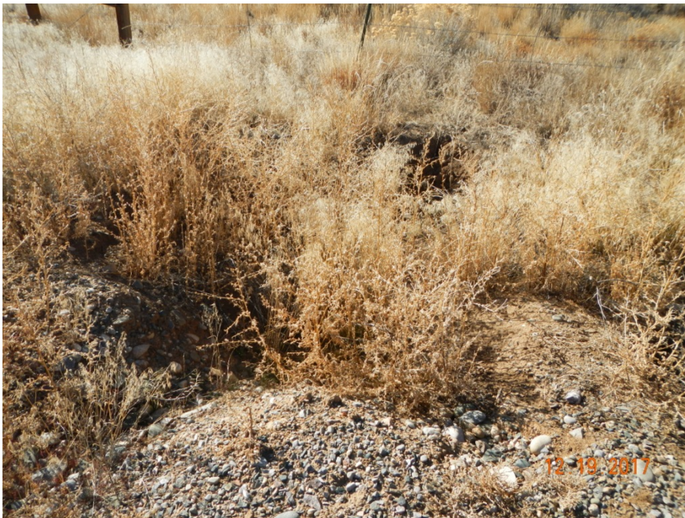
Photo 4. View of area where concentrated stormwater flows off of the southwestern corner of the well pad and tunnels through the interim reclamation area.
