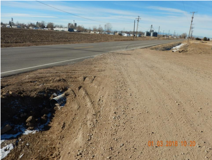
Photo 1. Photo taken from the entrance of location off CR90, facing West. Operator has installed a culvert along the bar ditch. Operator has installed gravel but may not be a sufficient tracking pad device by itself.
