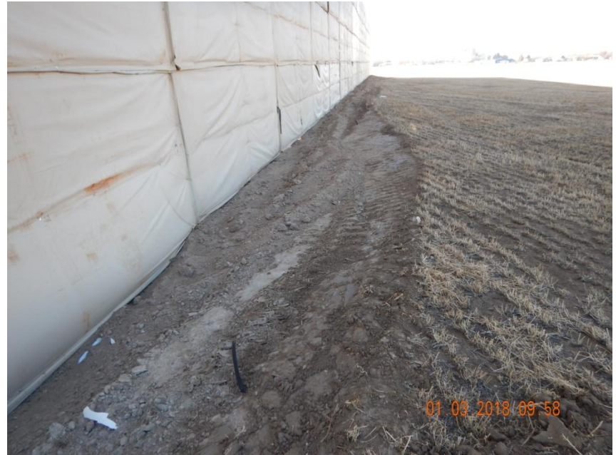
Photo 2. Photo taken from the cut slope of the northern location, facing West. Operator has failed to install stormwater BMPs per Rule 1002.f.(2).
