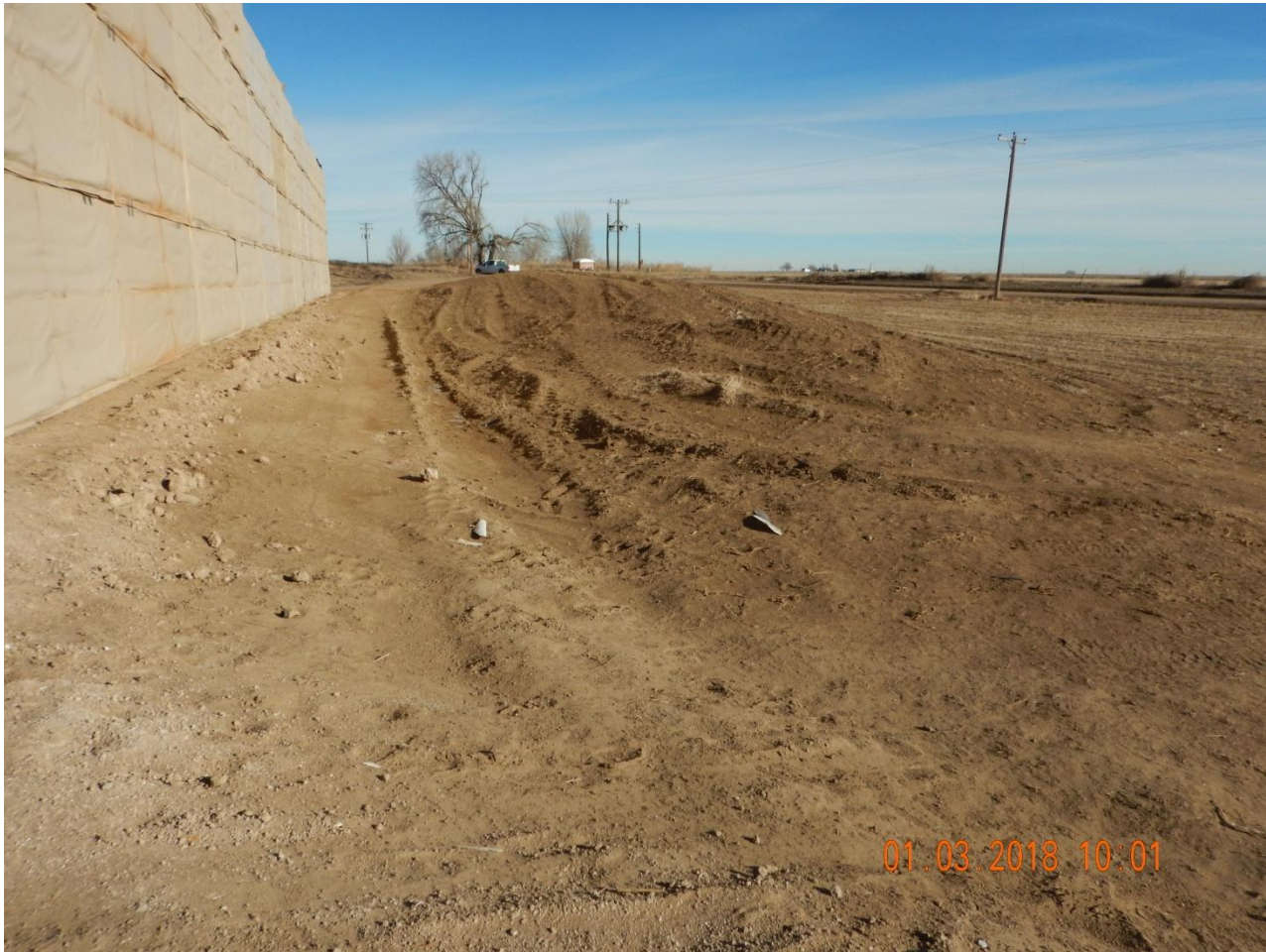
Photo 5. Photo taken from the eastern location, facing North. See comments under Photo 2. Topsoil stockpile stored along the eastern perimeter and appears to be temporarily stabilized with equipment tracking. Operator needs to stabilize topsoil stockpile for long-term stabilization.
