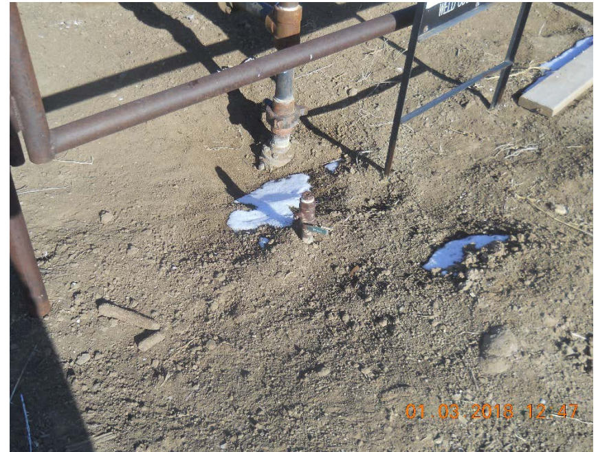
1" steel unused/unmarked riser at wellhead
