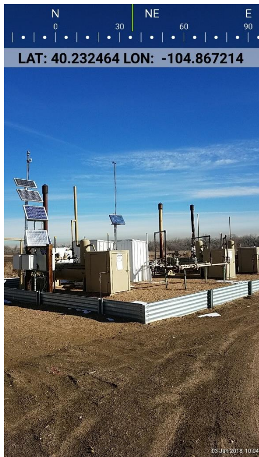
Photo 4 Separators and gas meter runs
