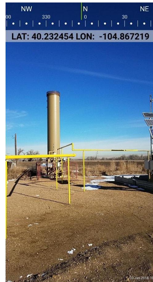
Photo 3 Emission control burner
