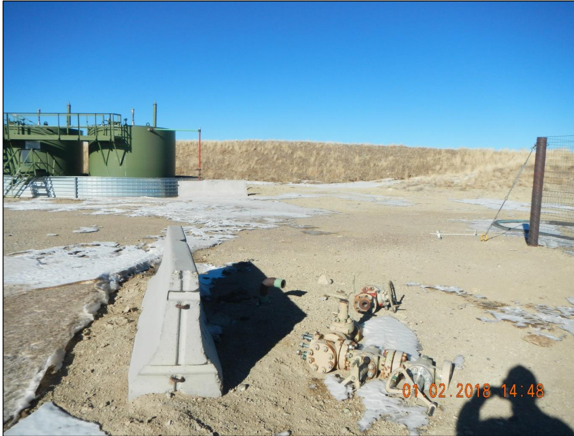
Unused equipment and 2" riser unmarked, no plug, valve, and no lock out tag out.
