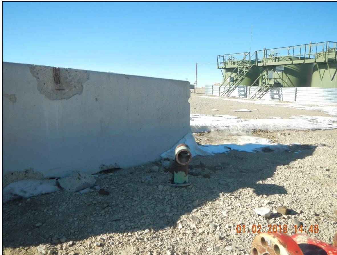
2" riser unmarked, no plug, valve, and no lock out tag out.
