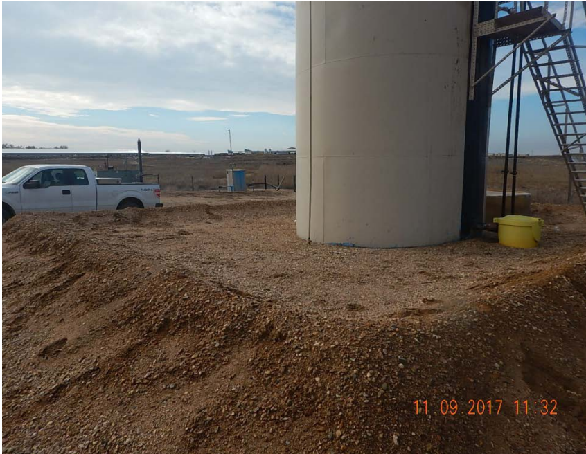
Photo 1: Location, looking SW
