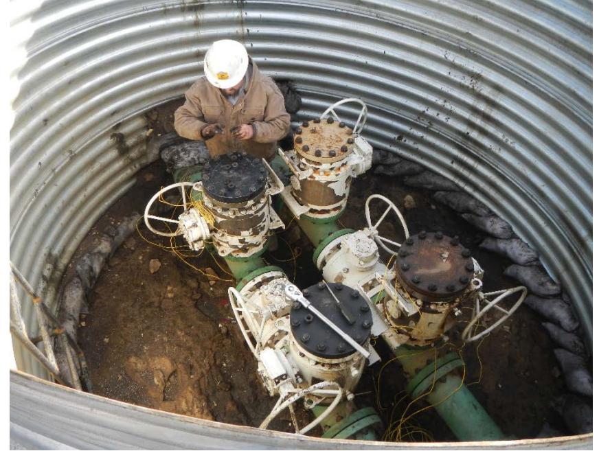
PW line being re-capped in valve can
