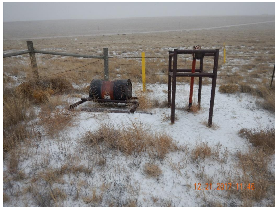
Photo 4: Photo taken from the south end of the location, facing southwest. Photo shows pipe riser and trash debris (barrel scraper, can be considered unused equipment) remaining on the location.
