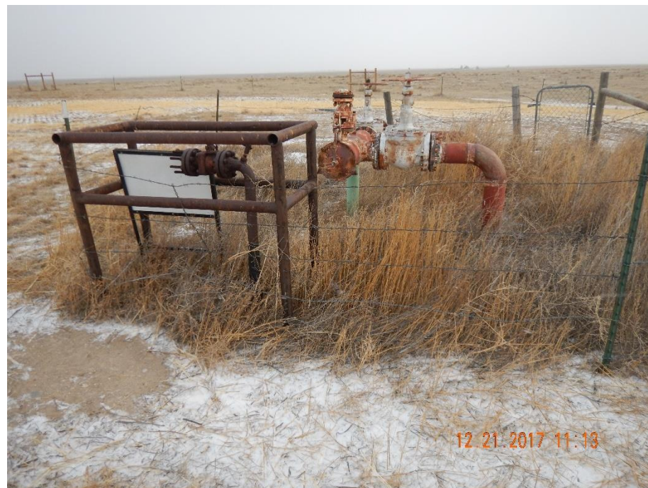
Photo 6: Photo taken from the location, facing east. Photo shows two (2) pipe risers remaining on the location. Riser seen in cage to the left is pipe seen in photo 4 and 5. Equipment to the right possibly belongs to DCP as a DCP flag was observed at its base.
