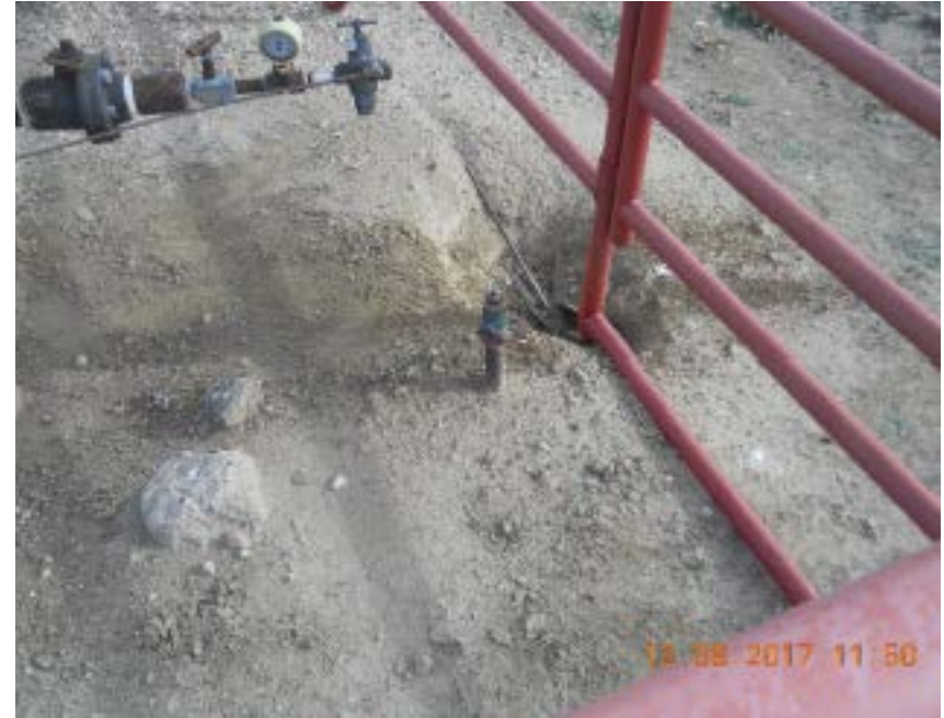
1" steel riser at wellhead from previous inspection
