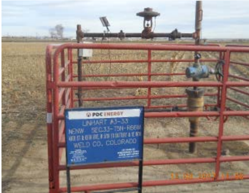
Wellhead looking east from previous inspection
