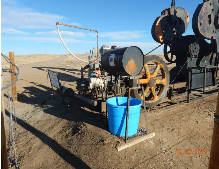
Photo #3 – Day tank with secondary containment.
