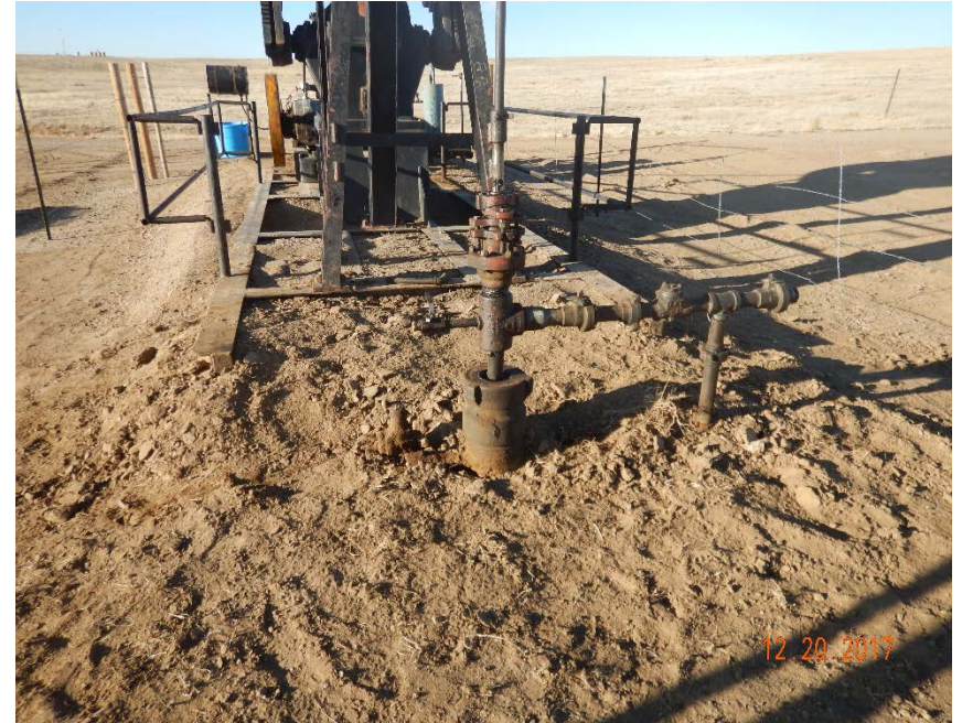
Photo #4 – Improved conditions at wellhead.
