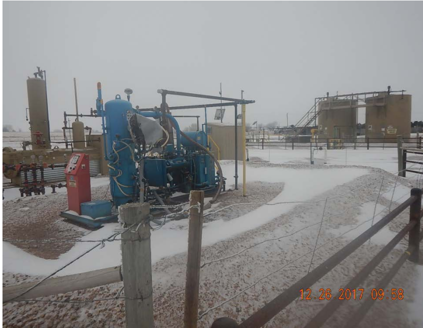
Photo 1: Location, looking SW
