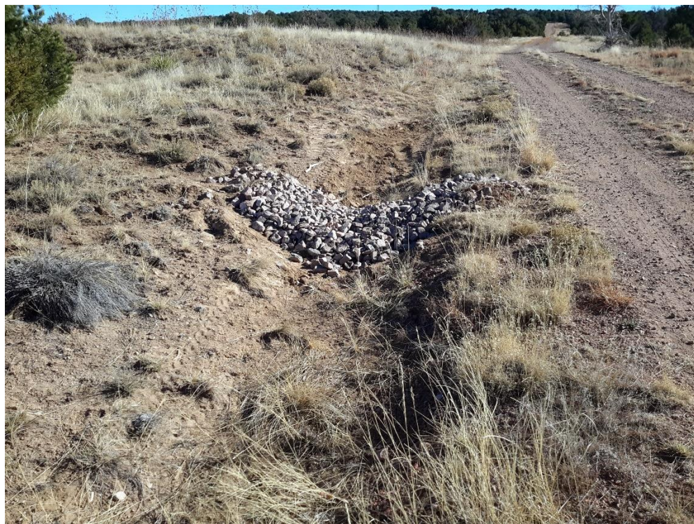
Loose Rock Check Dam: Between State 2W and State 3W northeast side of access road
