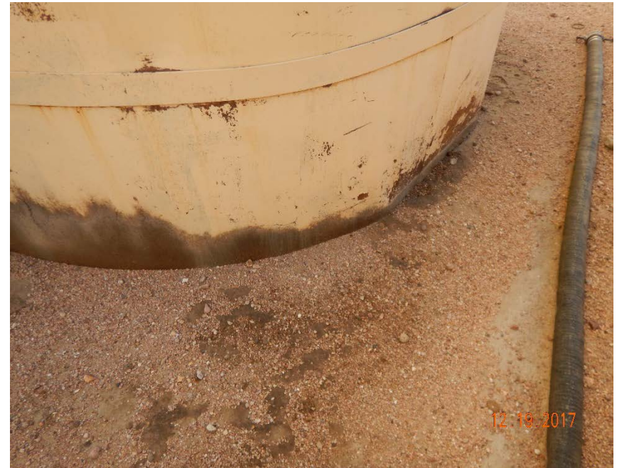
Photo #26 - Localized accumulations of oily waste beneath produced water ASTs and associated equipment (3).
