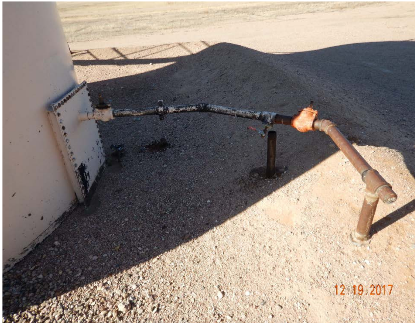
Photo #7 - Localized accumulations of oily waste underlying valves and equipment at crude oil tank battery (4). Note abandoned flowline risers north of crude oil ASTs and shallow earthen berm.
