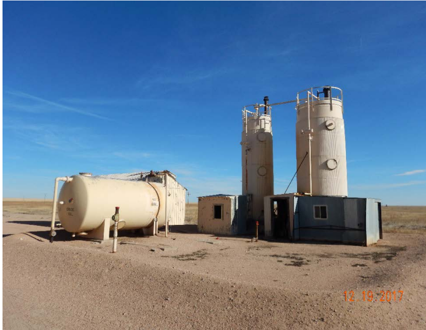
Photo #11 – Horizontal crude oil AST with VHT sheds located at SE corner of facility. Note shallow earthen berm.
