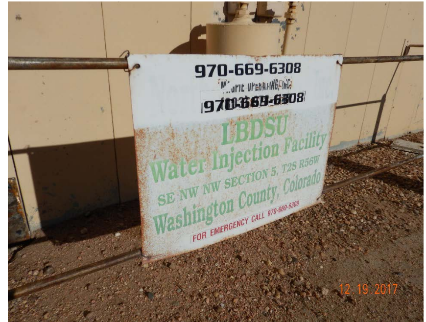
Photo #30 – Operator sign located on south side of main injection building. Note that operator name is illegible.
