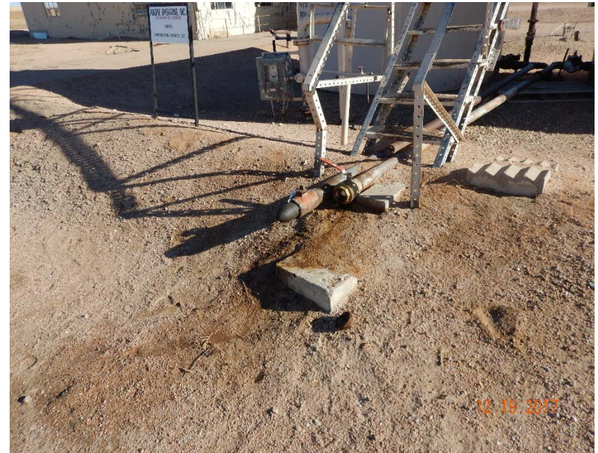
Photo #2 – Stained soil at crude oil AST loadout. Note shallow earthen berm.
