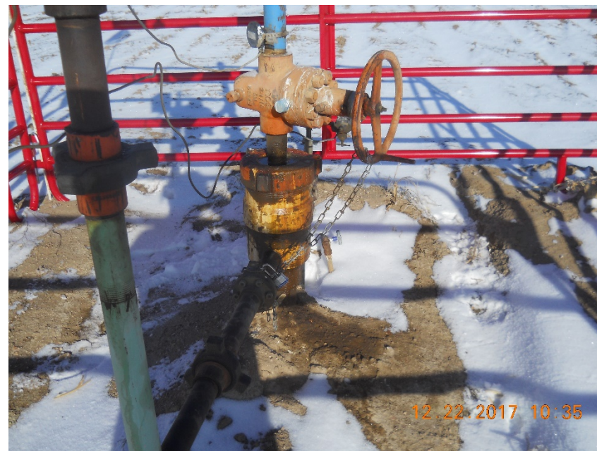
Stained soil under master valve. Appears to be leaking/have leaked from wellhead packing
