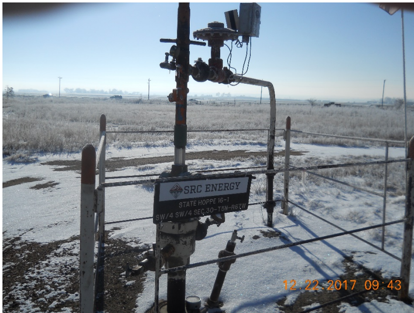
Wellhead looking south, no emergency contact information. No MIT on file, no recorded production since Nov. 2015
