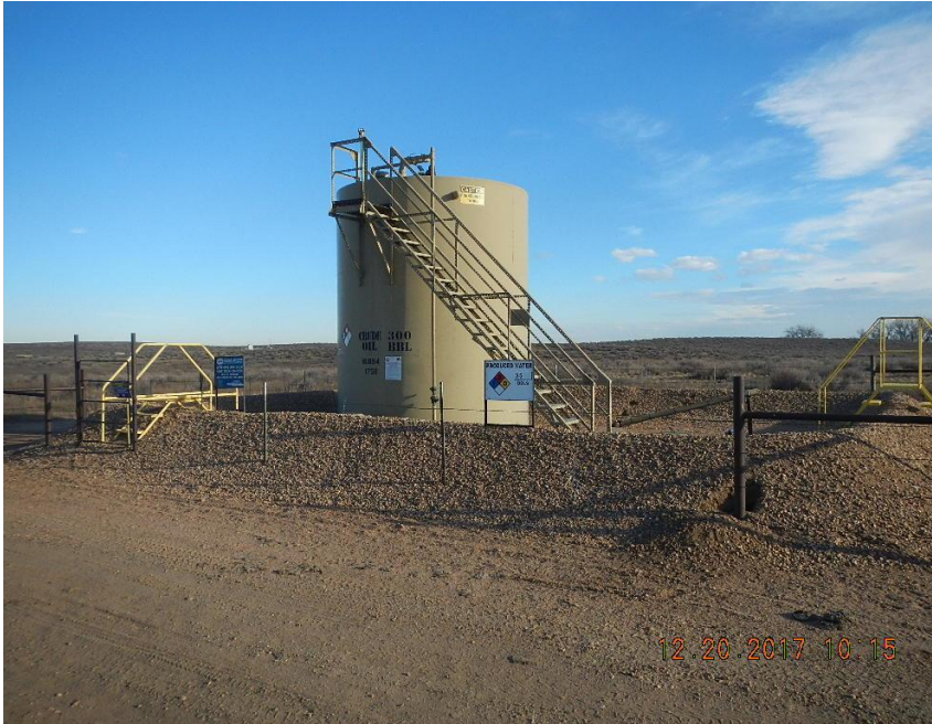
Photo 1 Tank Battery from West
