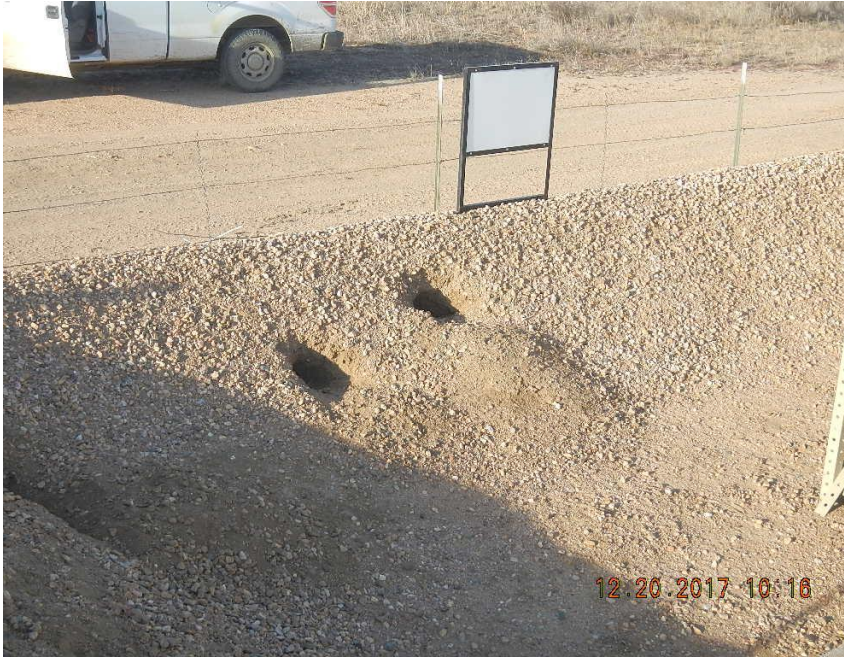
Photo 3 Burrow in berm from southeast
