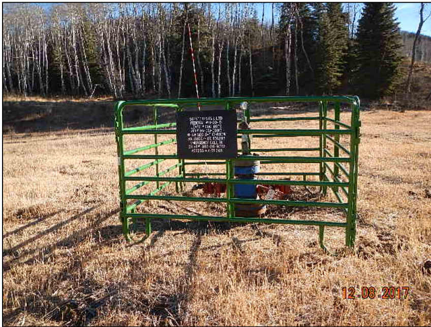
Photo 1. Vegetation has been removed from around the wellhead.
