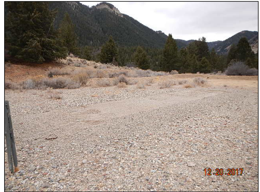
Photo 2. Concrete pad and pumpjack parts have been removed.
