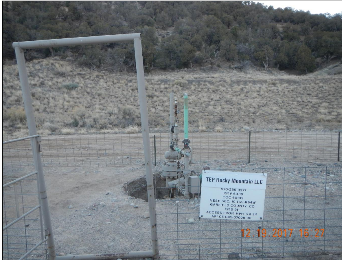
Cellar dug around well head of RMV 63-19
