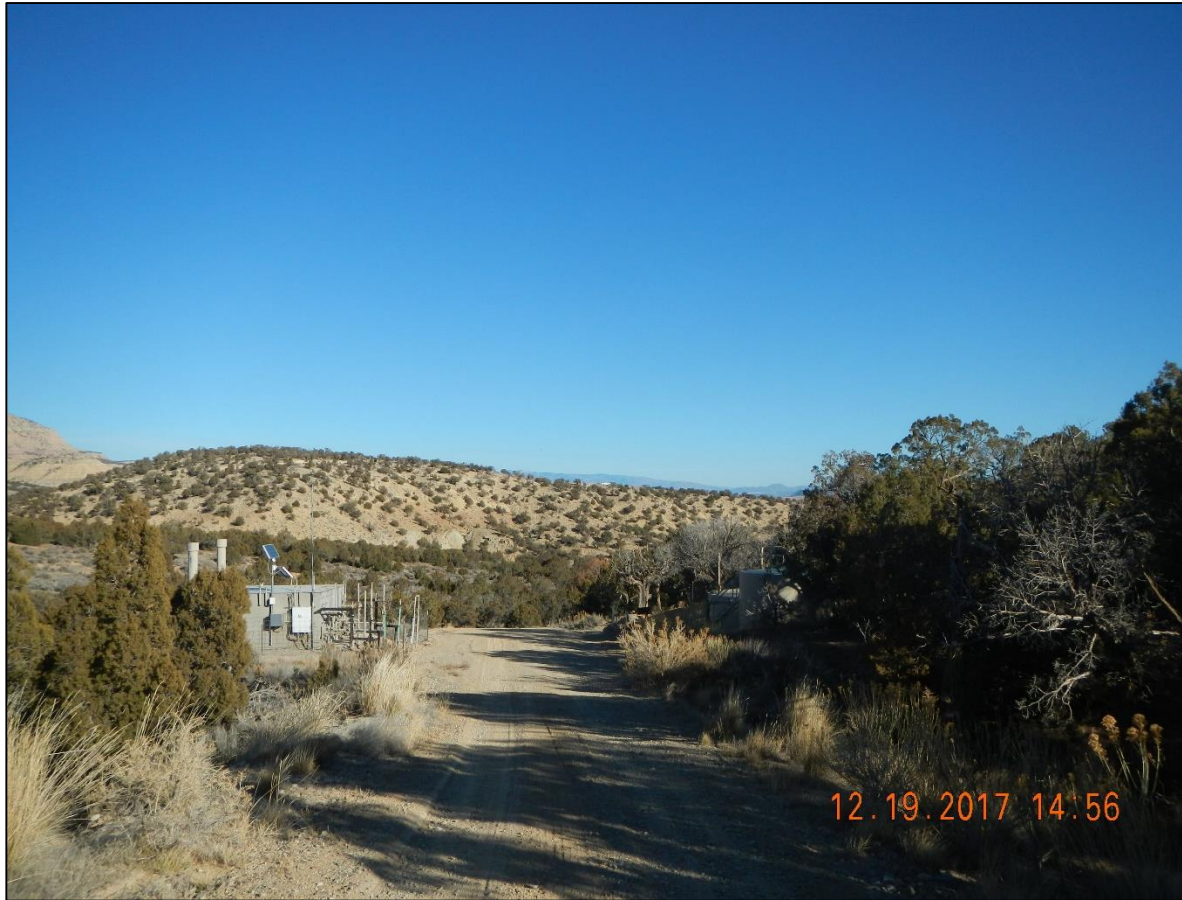
Separators and tank battery.
