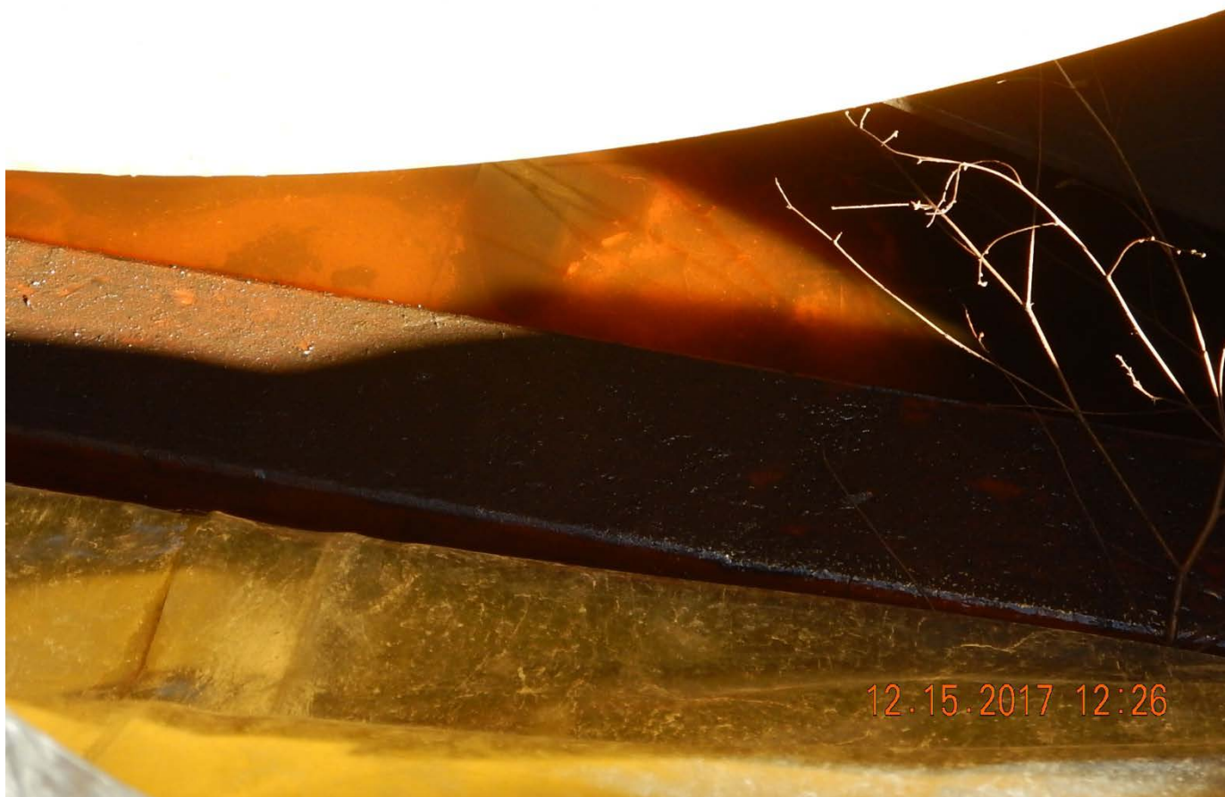
Fuel tank secondary containment. Containment is approximately half full with hydrocarbon/water mix.
