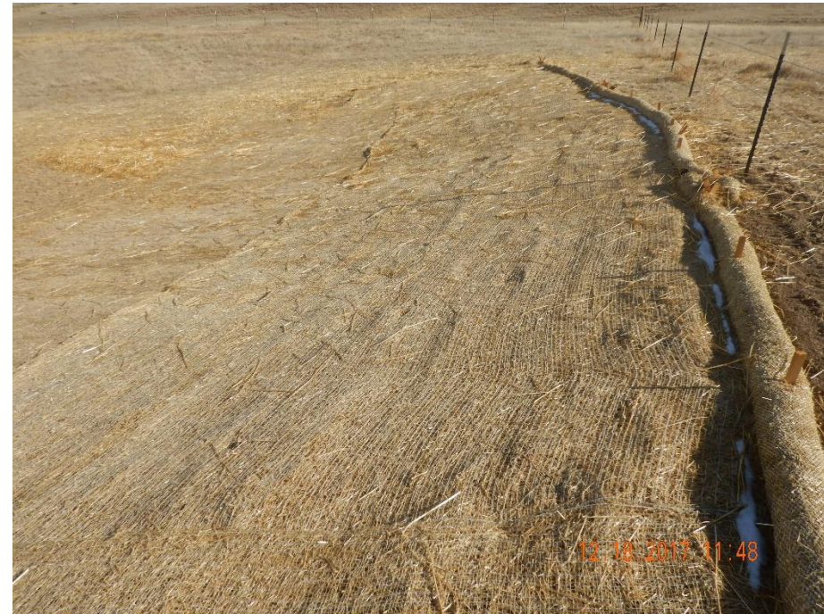
Photo 6: Photo taken southwest corner of the well location, facing east. Photo shows well pad appears to have been recontoured/regraded, seeded and stabilized w/ matting.
