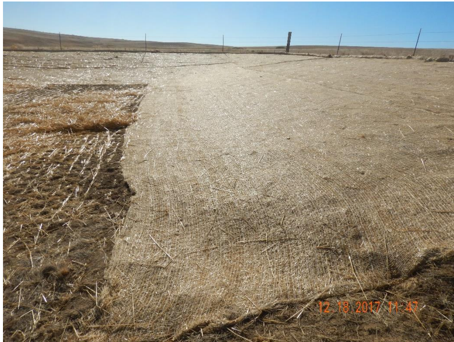
Photo 5: Photo taken southwest corner of the well location, facing south. Photo shows well pad appears to have been recontoured/regraded, seeded and stabilized w/ matting.
