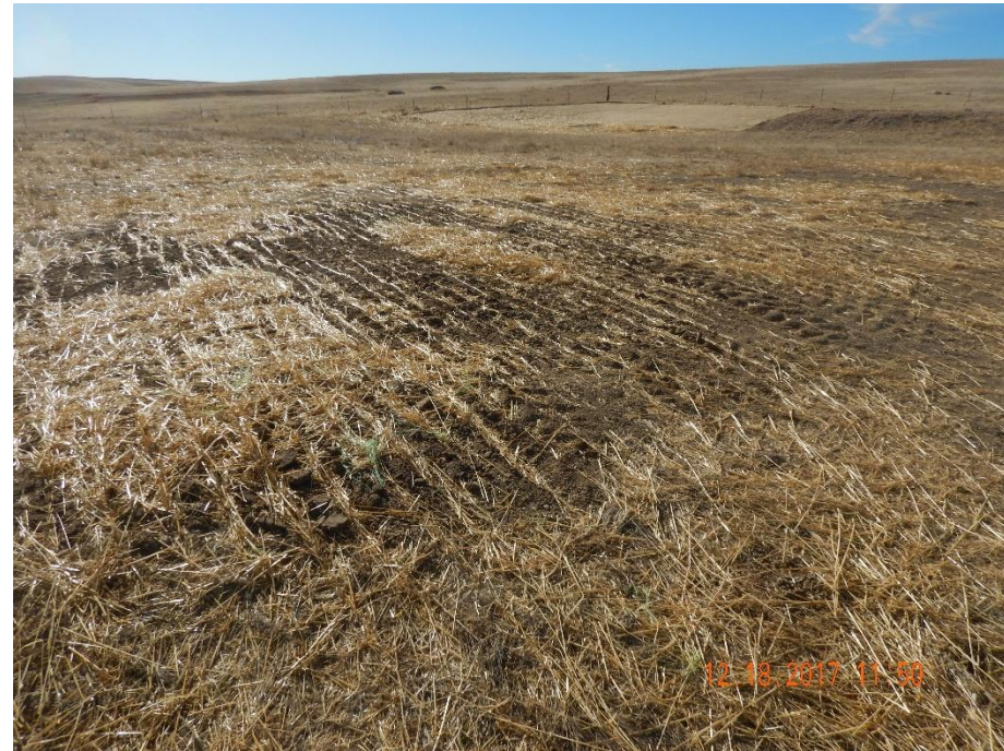
Photo 8: Photo taken from well location, facing southwest. Photo shows gravel has been removed from well location and area appears to have been reseeded and crimped with straw for stabilization.
