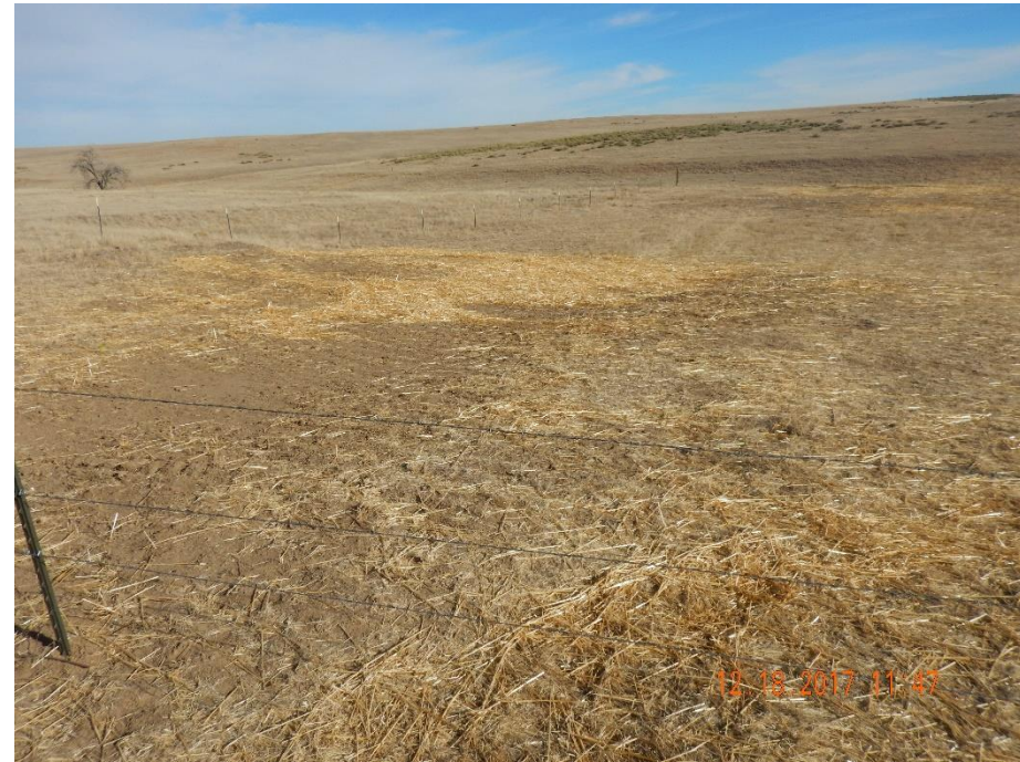
Photo 2: Photo taken from the west end of the well pad location, facing east. Photo shows well pad appears to have been recontoured/regraded, reseeded and crimped with straw for stabilization.
