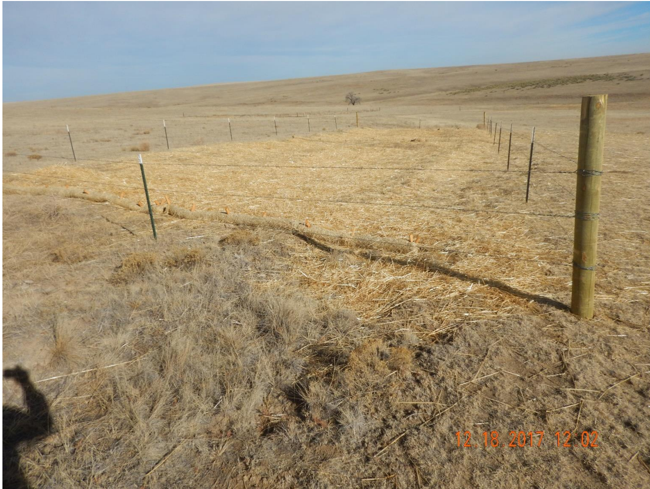
Photo 11: Photo taken from the access road, facing east. Photo shows area of access road that appears to have been regraded, seeded and crimped with straw for stabilization.
