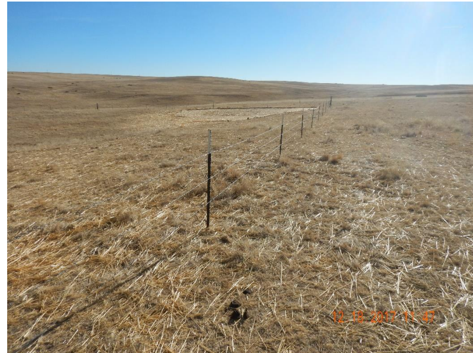
Photo 4: Photo taken from the west end of the well pad location, facing south. Photo shows well pad appears to have been recontoured/regraded, reseeded and crimped with straw for stabilization.
