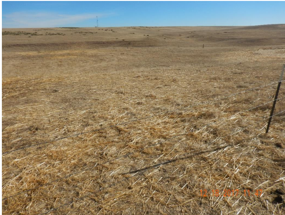
Photo 3: Photo taken from the west end of the well pad location, facing southeast. Photo shows well pad appears to have been recontoured/regraded, reseeded and crimped with straw for stabilization.
