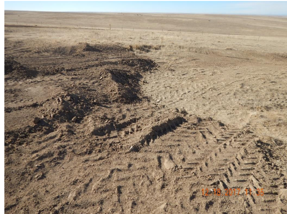
Photo 6: Photo taken from the fenced area of the northern spill area, facing west. Photo shows areas that appear to have been recontoured/regraded and additional topsoil brought in. Areas do not appear to have been seeded and stabilized; reclamation activities do not appear to be complete in accordance to the corrective action. Corrective action and date will remain applicable until corrective action has been addressed.
