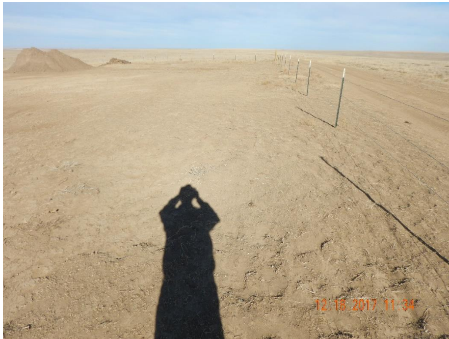
Photo 1: Photo taken from within the fenced area of the northern spill area, facing north. Photo shows areas that appear to have been regraded/recontoured and additional topsoil brought in. Areas do not appear to have been seeded and stabilized; reclamation activities do not appear to be complete in accordance to the corrective action. Corrective action and date will remain applicable until corrective action has been addressed.
