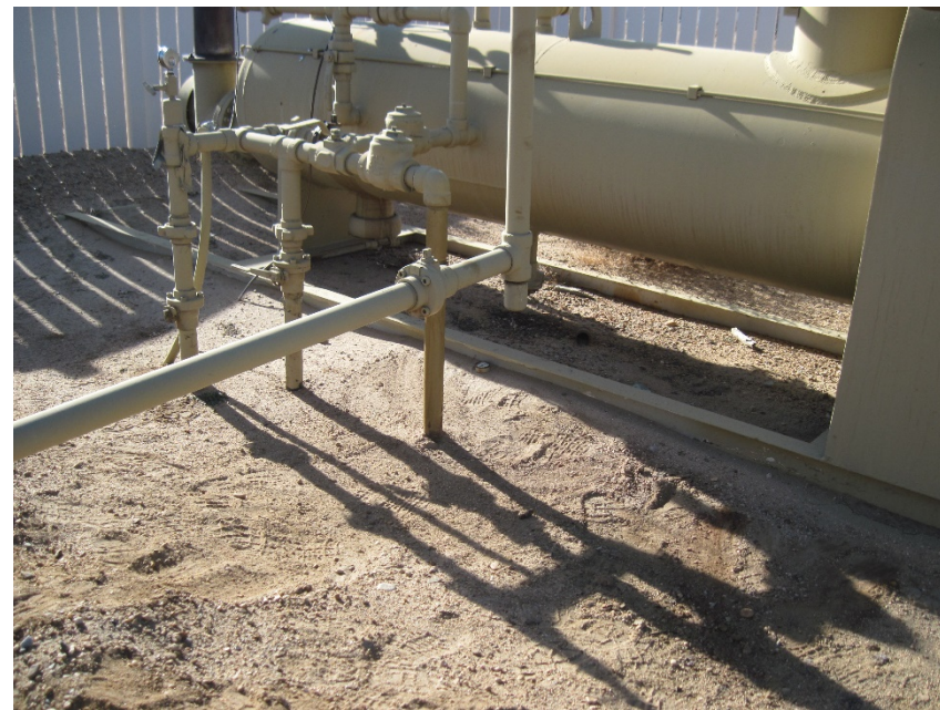
Repaired leaking line on Seperator
