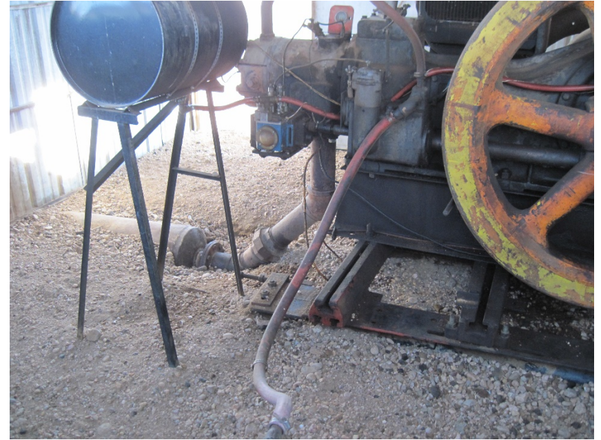
Pump jack house soiled dirt removed
