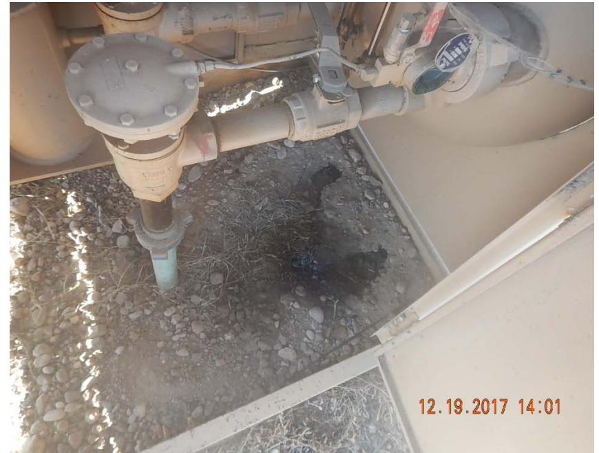
Photo 4: Stained soil in separator house
