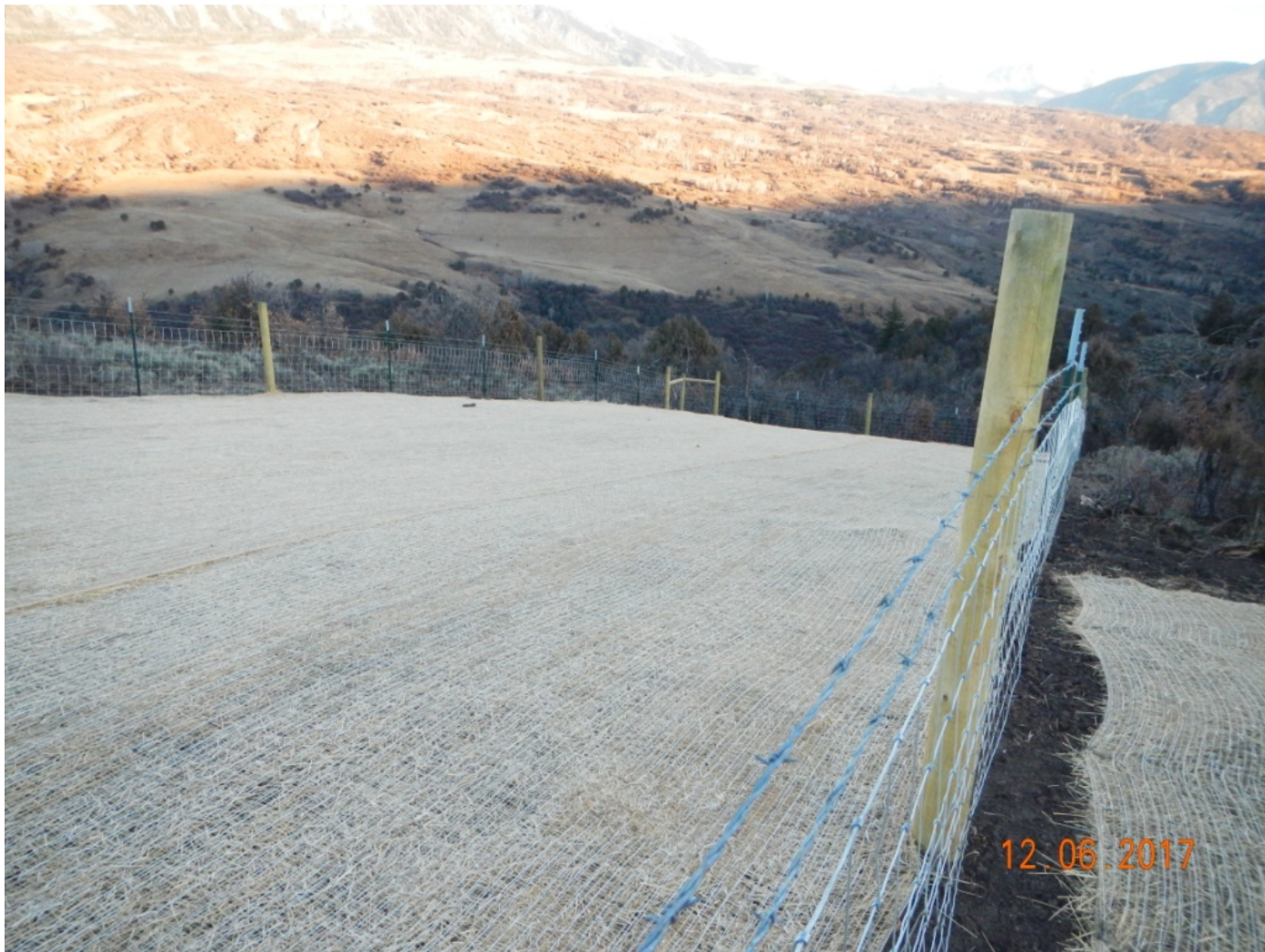
Photo 1. View of area recently reclaimed. From the southwester edge facing eastward. Showing erosion control blanket and fencing.
