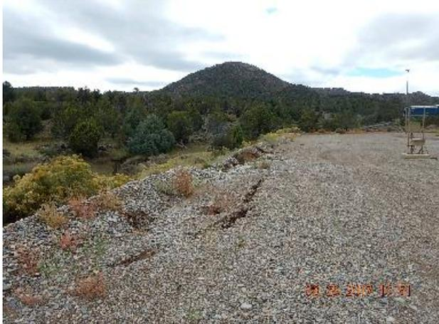
Photo 3: Separation in E fill slope. Previous inspection.
