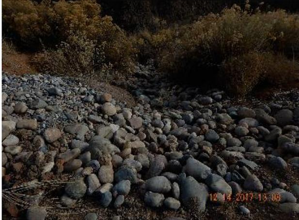
**Photo 7: Rock in the repair to the erosion channel on fill slope.**
