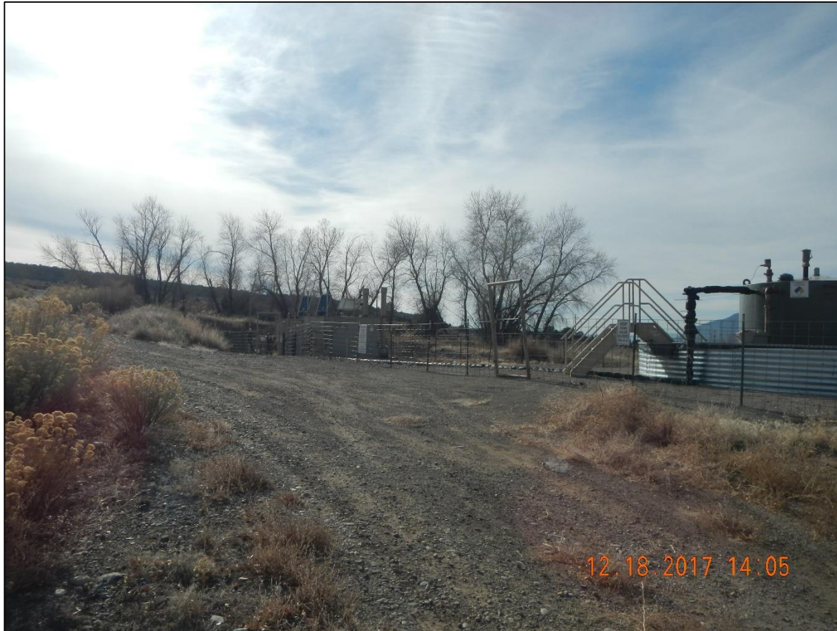
Separators and tank battery.
