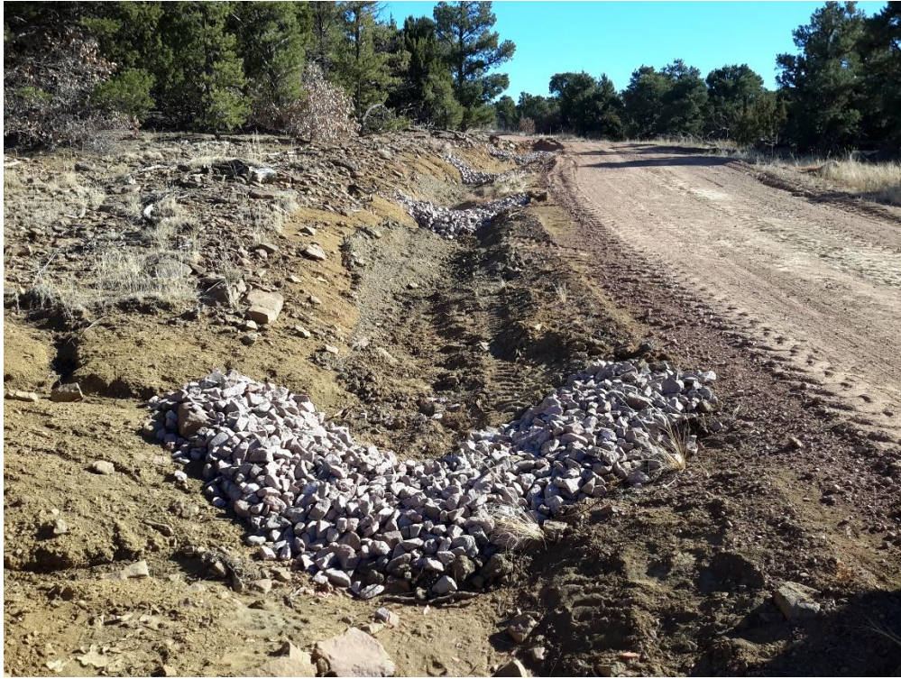
Loose Rock Check Dams: Between State 7W and State 9W northeast side of access road
