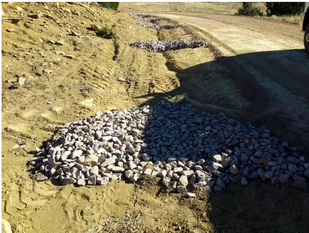
Loose Rock Check Dams: Between State 9W and State 10WB northeast side of access road
