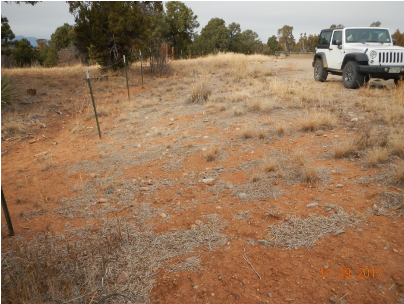
Photo 1. View of straw and area with documented erosion, appears to be functioning, but controls may not be sufficient. No clear whether the area was seeded.
