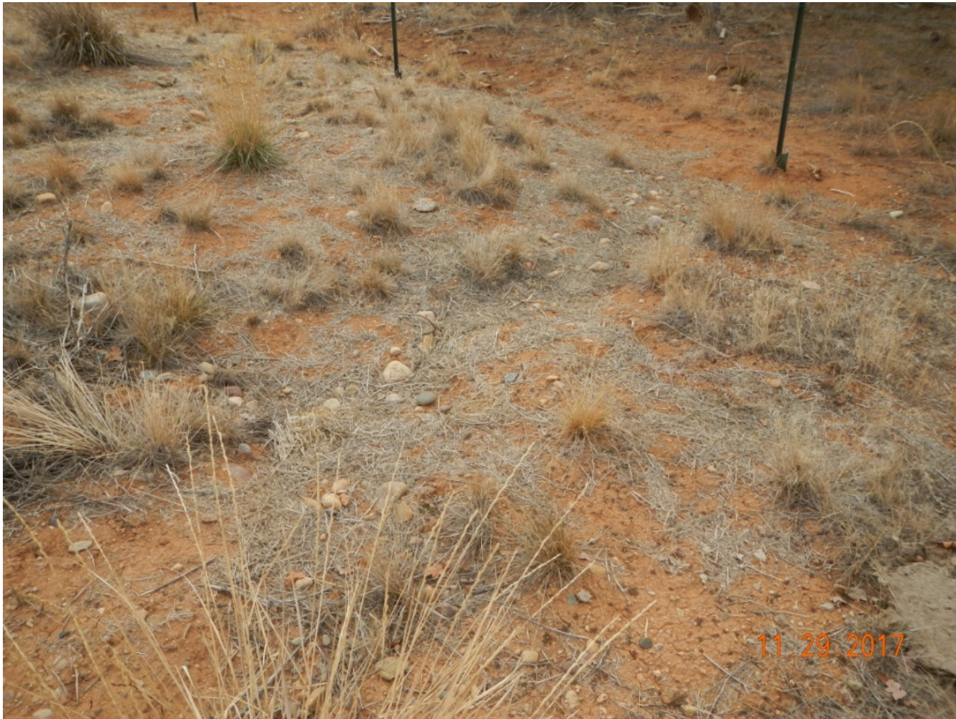
Photo 2. View of area where erosional channel has been filled and straw applied. Not clear whether it's been seeded.
