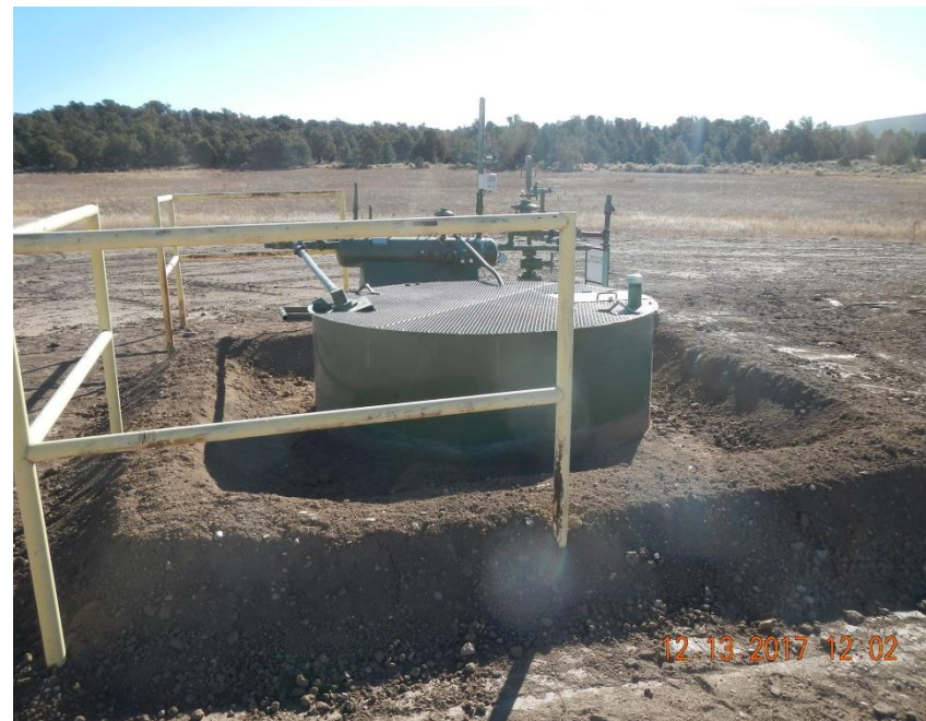
Secondary containment berm has been repaired.
