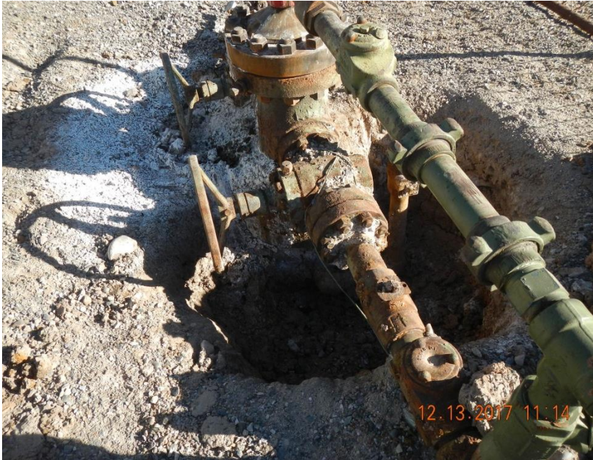
Alternate view of excavation near well head.
