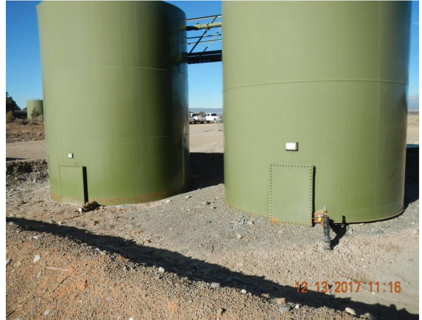
Secondary containment berm for tank battery has been repaired.
