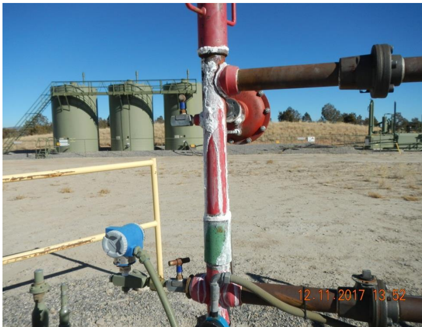
White residue on #147T well head.
