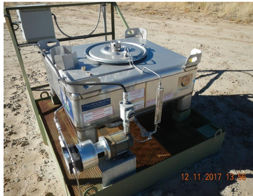
Chemical injection system for #19M well head with no label or placard.
