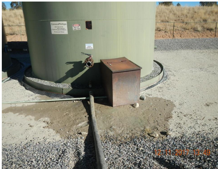
Release beneath truck load out valve.
