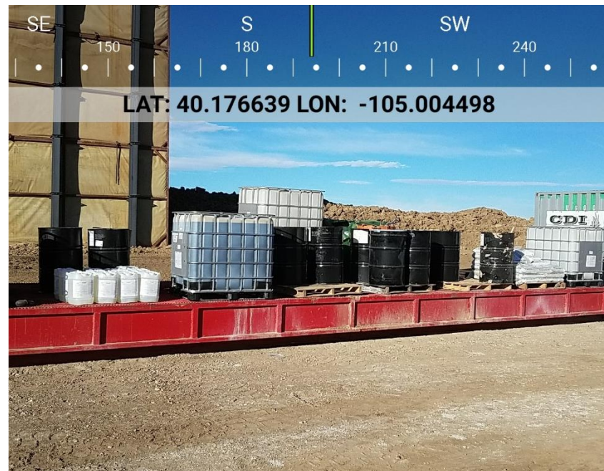
Photo 10 Secondary containment below fluid chemical storage from east
