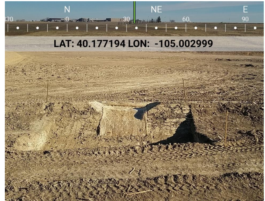
Photo 14 Storm water settling area east of location entrance.
