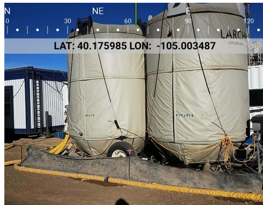
Photo 8 Secondary containment on waste management and potable water
