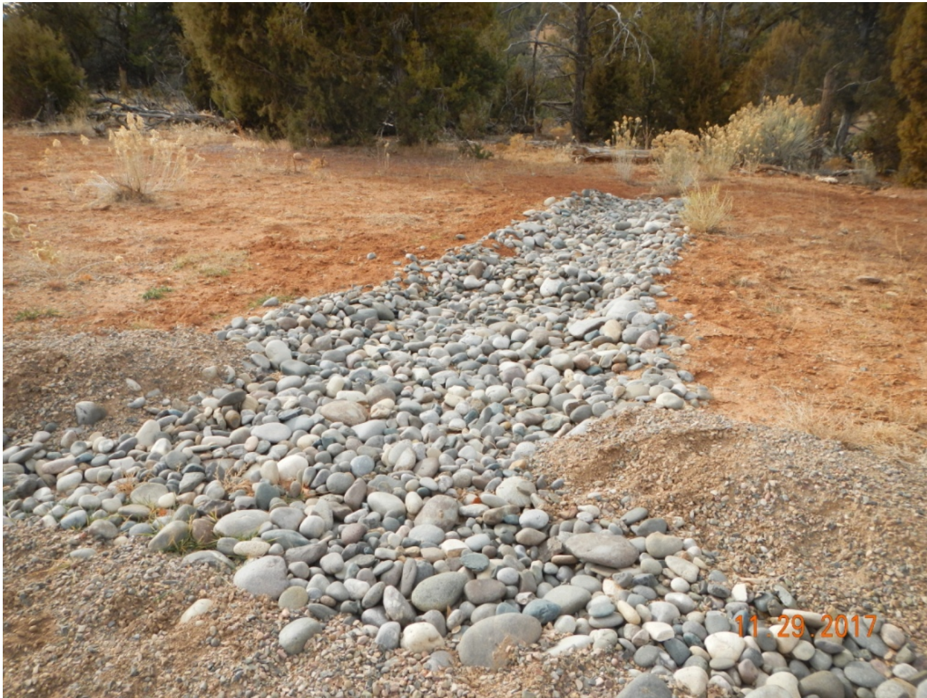
Photo 3. View of cobble run-down in the western portion of the project area.
